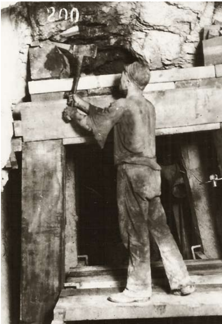
FIGURE 12.7: Nearly 10,000 miles of mine tunnels threaded beneath Butte Hill alone. To keep the tunnels from collapsing, workers placed massive timbers every few feet.
