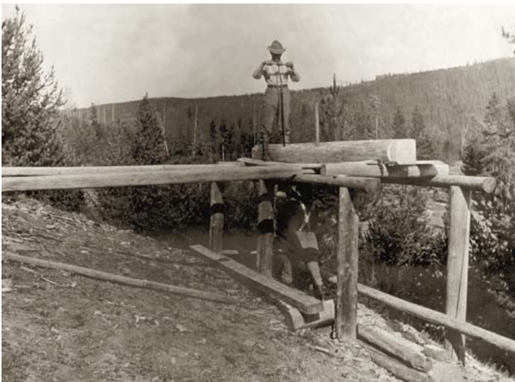
FIGURE 12.5: A whipsaw allowed two men to cut planks from logs. They dug a pit, or built a tall structure like this one, and secured the log so it would not roll. Then, with one man on top and one below, they drew a long, two-handled saw up and down through the length of the log.
