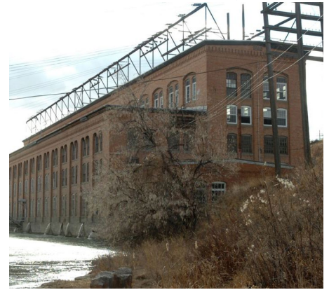
The Rainbow Dam Powerhouse as it currently appears from the downstream side, ready to assume a new role in Great Falls's ongoing development.
