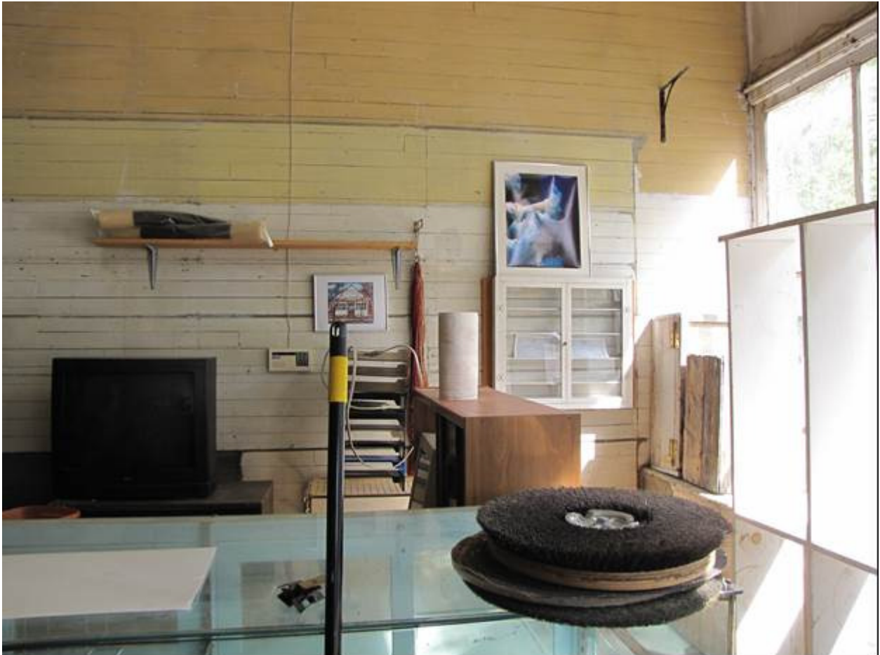
MT_LewisAndClarkCounty_DorseyGroceryAndResidence_0013. Grocery, interior, east wall with silhouette of original shelving, view to E.
