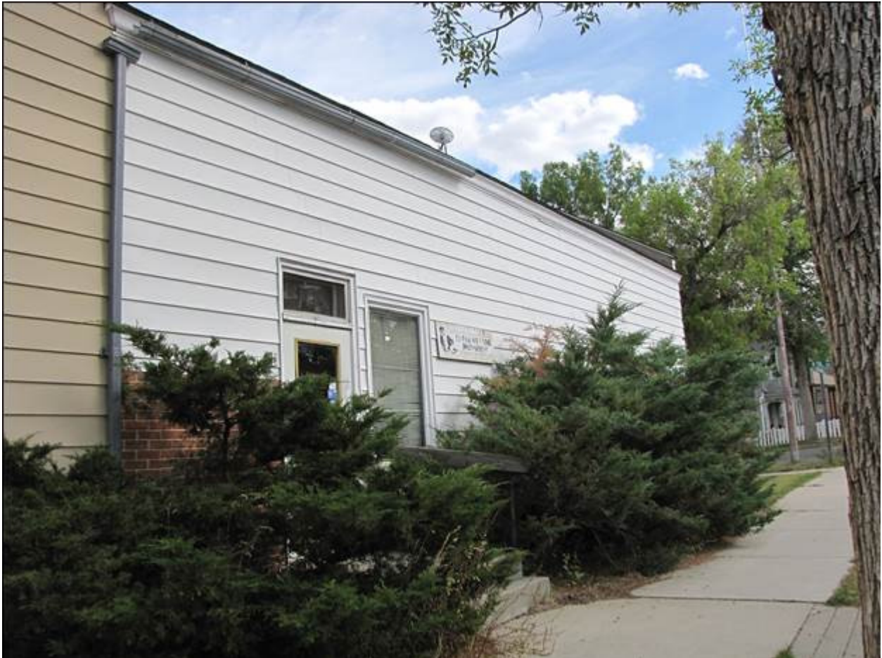
MT_LewisAndClarkCounty_DorseyGroceryAndResidence_0005. Grocery, west wall, view to SE.
