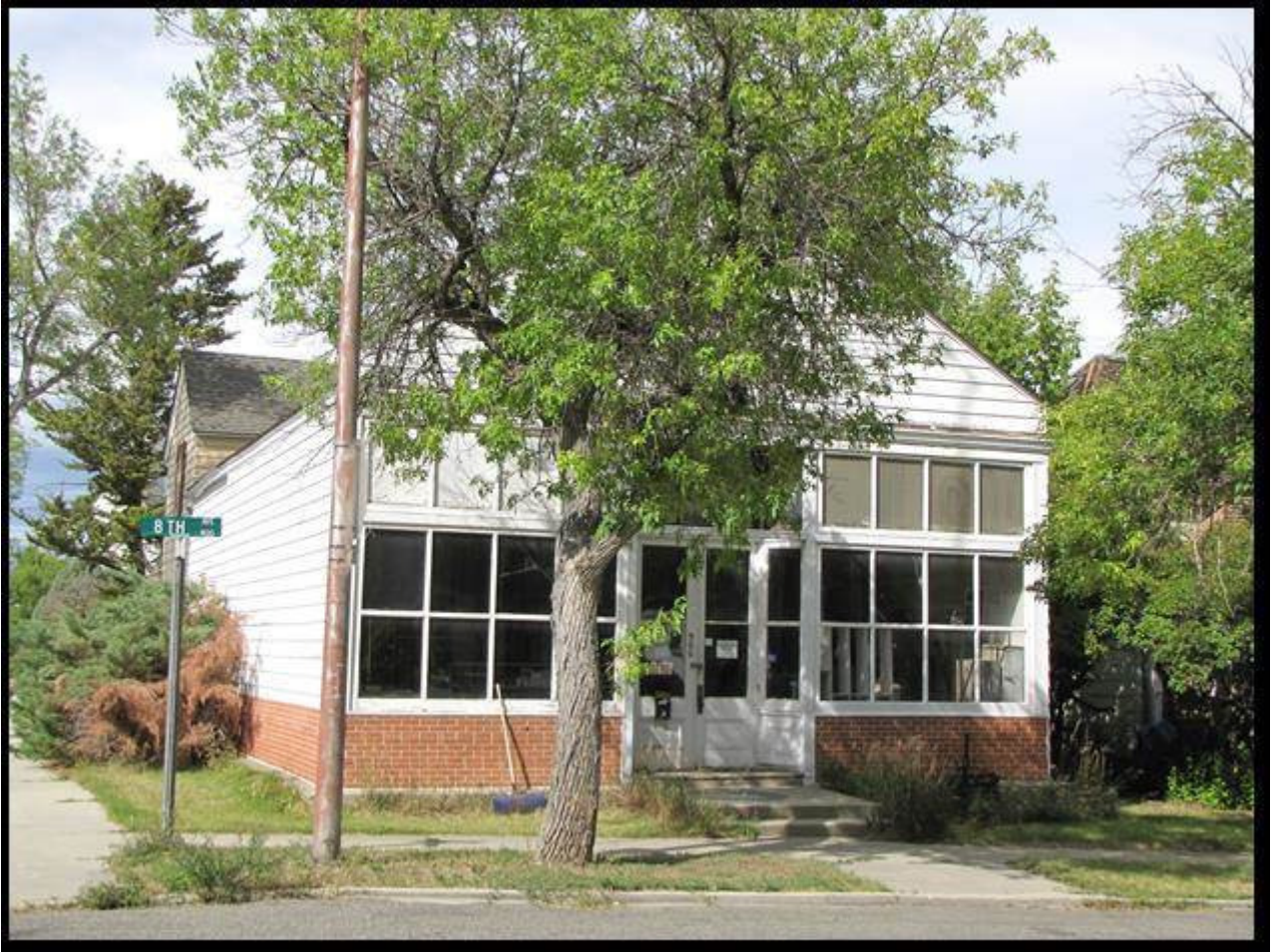
MT_LewisAndClarkCounty_DorseyGroceryAndResidence_0003. Grocery, façade (south) and west wall, view to N-NE.
