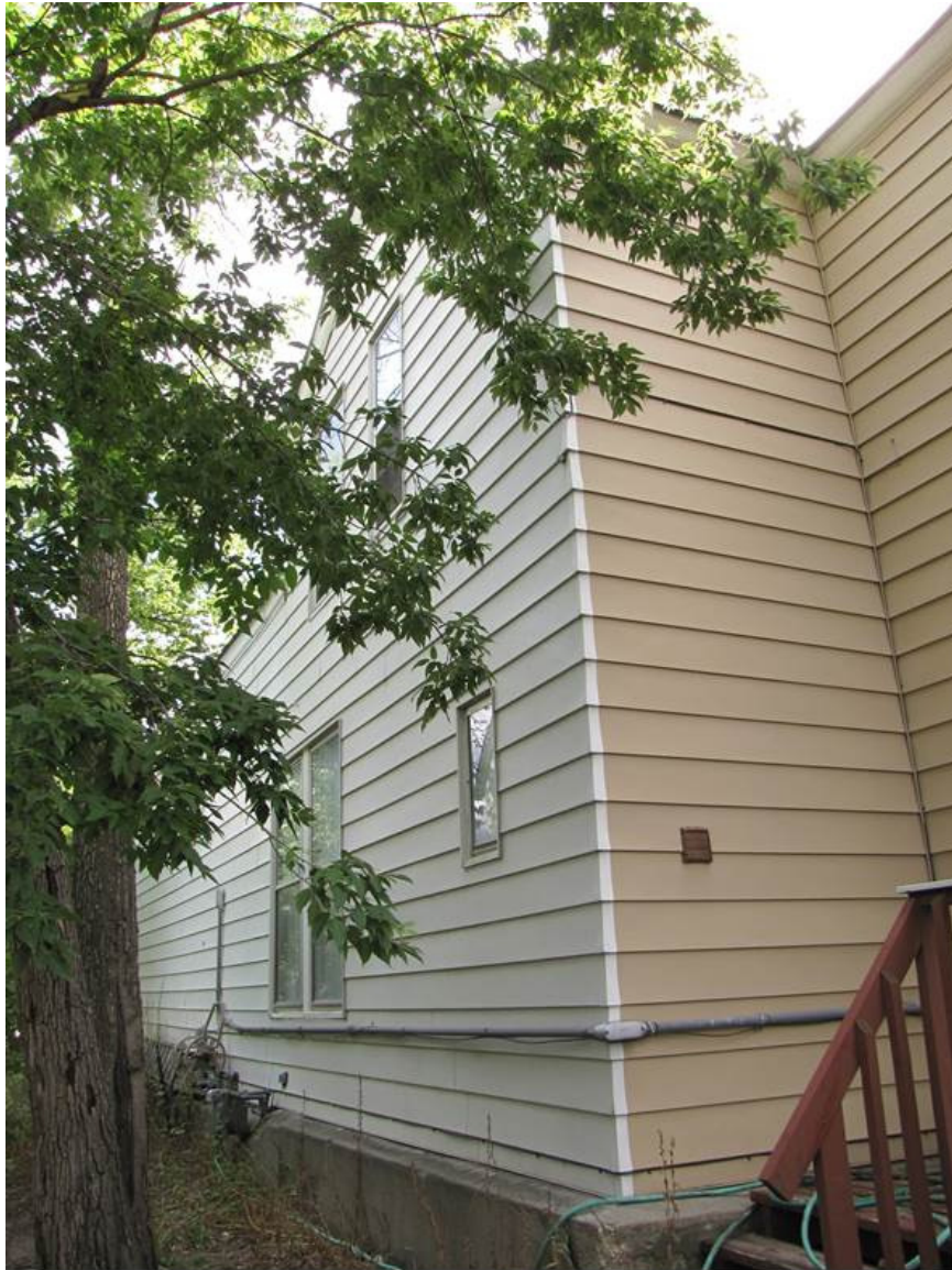
MT_LewisAndClarkCounty_DorseyGroceryAndResidence_0010. Residence, east wall, view to SW.
