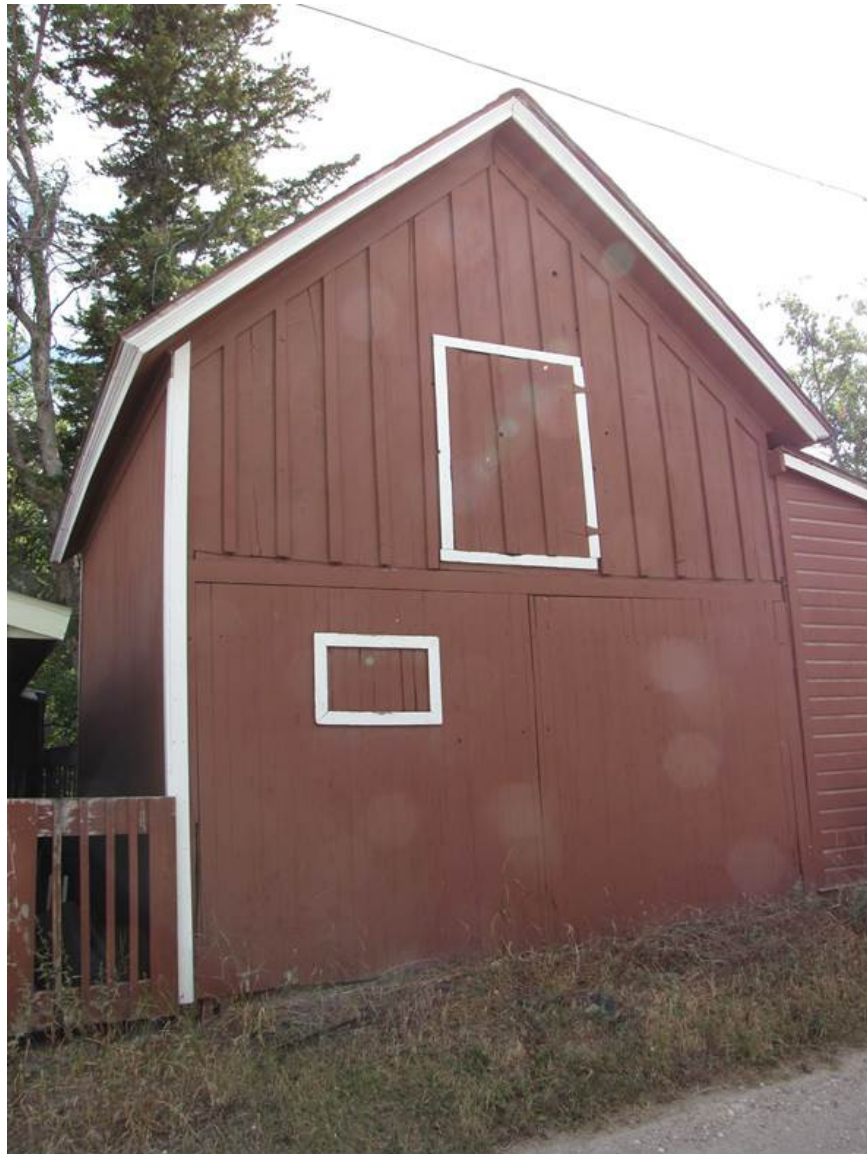
MT_LewisAndClarkCounty_DorseyGroceryAndResidence_0022. Garage/Carriage House, north and east walls of carriage house component, view to S-SW.
