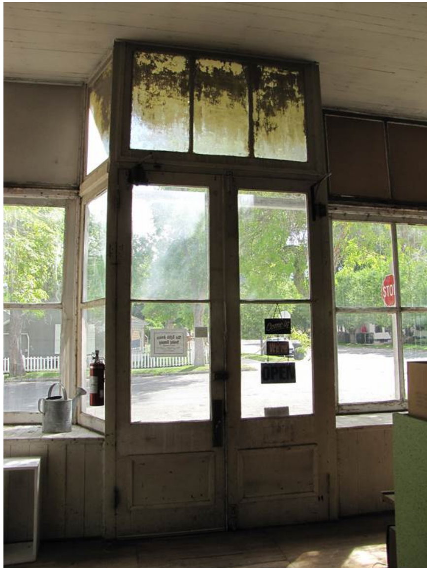
MT_LewisAndClarkCounty_DorseyGroceryAndResidence_0012. Grocery, interior, entry detail, view to S.
