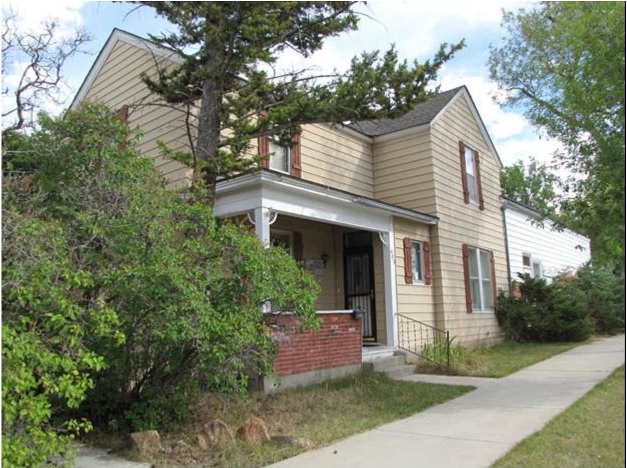
MT_LewisAndClarkCounty_DorseyGroceryAndResidence_0008. Residence, façade (west) and north walls, view to SE.
