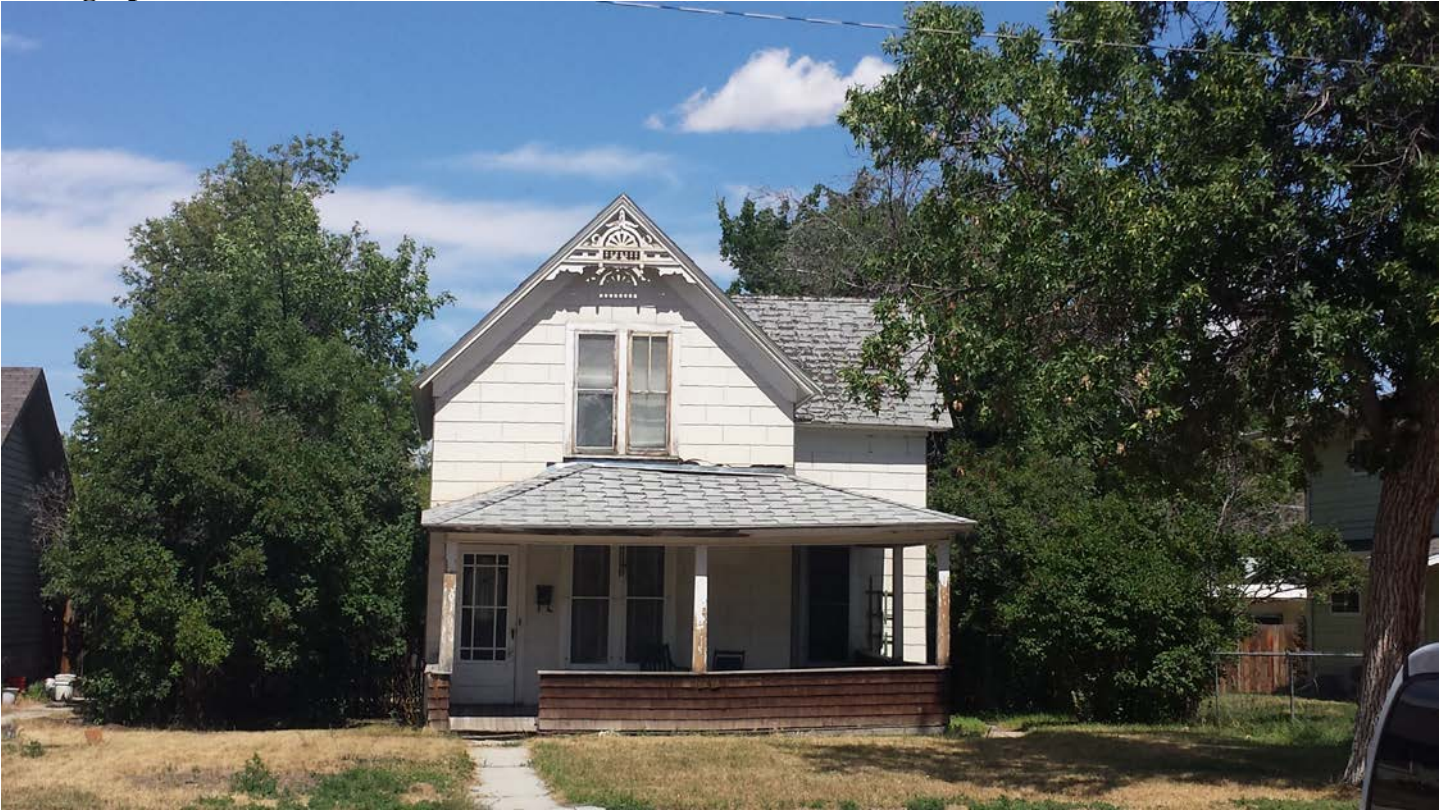
Knott Residence South Façade, facing north 7/24/15 Photo by Anthony Wood
