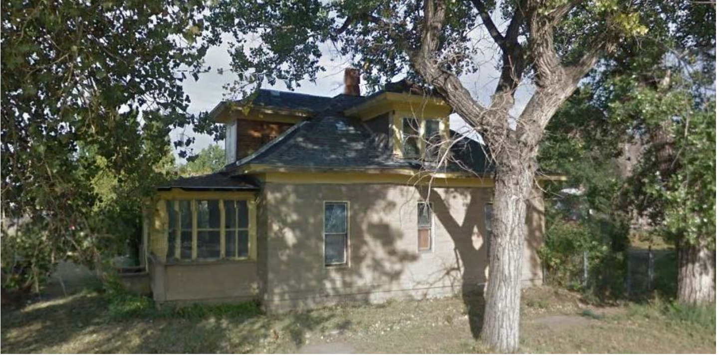
Dan Hurt House West elevation, facing east 8/13/15, (Google Earth Photo)
