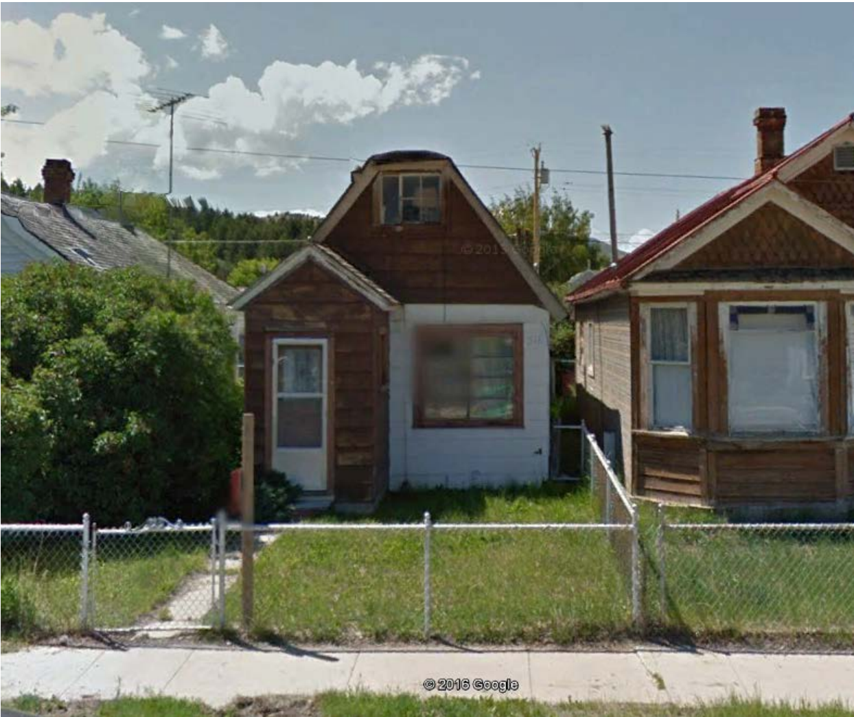
Frank and Sarah Q. Walker Residence 516 Spruce Street Anaconda, MT East Façade, view West Photograph from Google Earth
