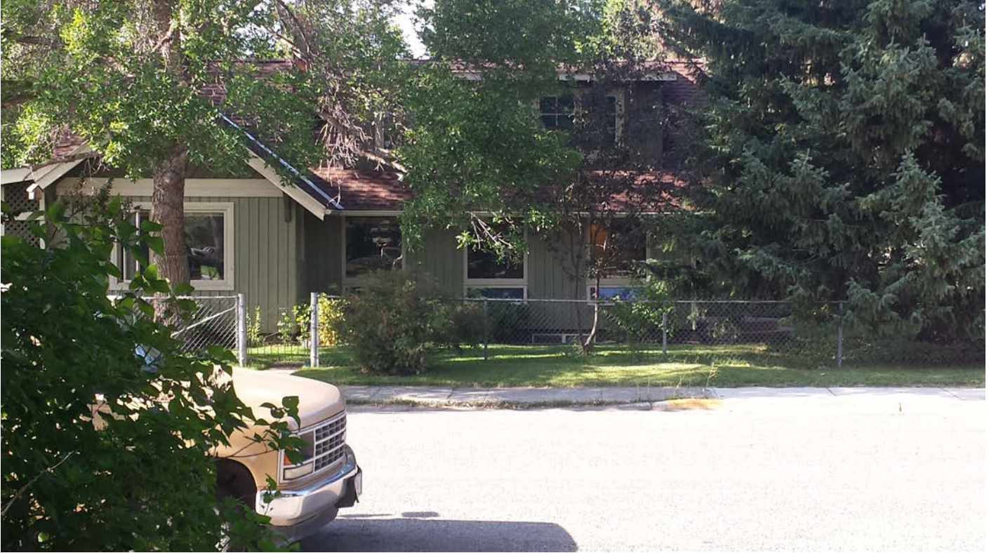
Oswald and Ada Smith House 503 North Bozeman Avenue South Elevation, facing North Photographed by Anthony Wood 8/1/16
