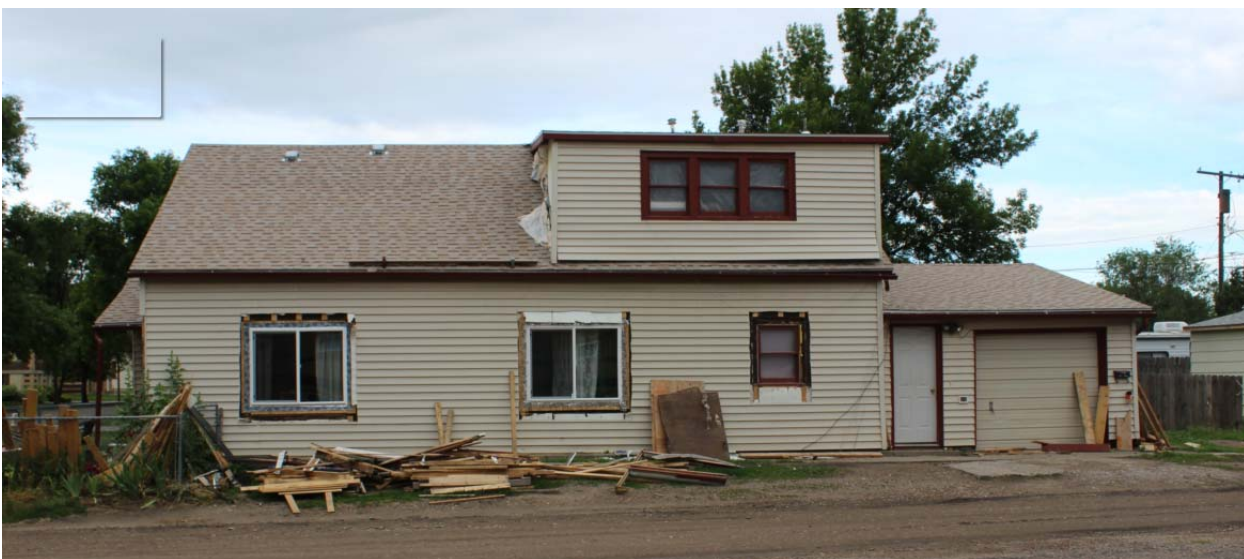
731 4 th Street, East Elevation, view W
