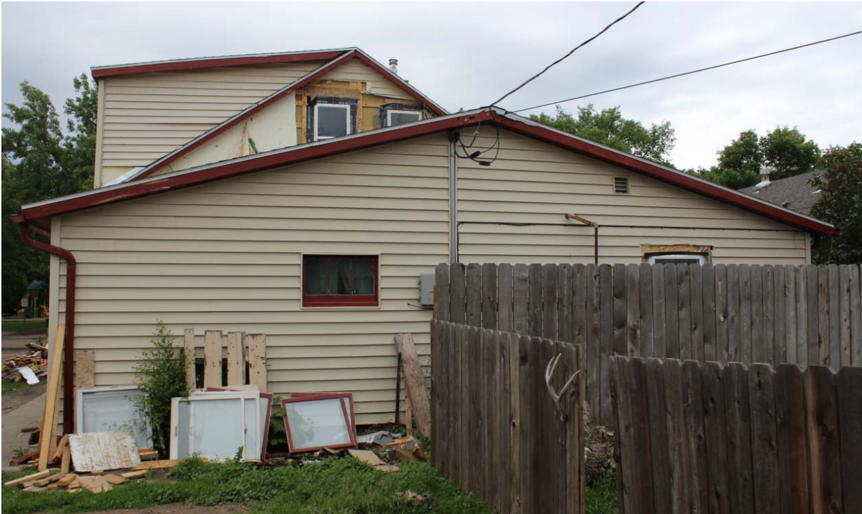
731 4 th Street, North Elevation, view S
