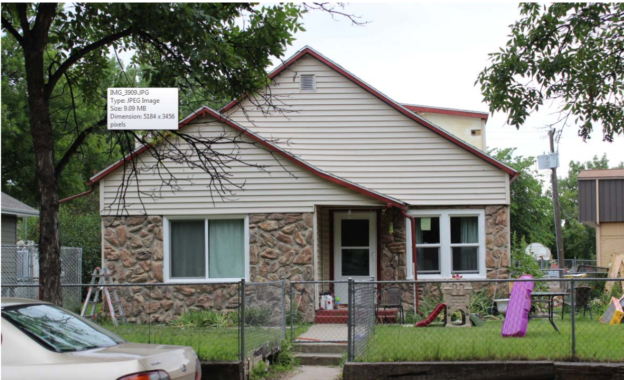
731 4 th Street, South Façade, view N
