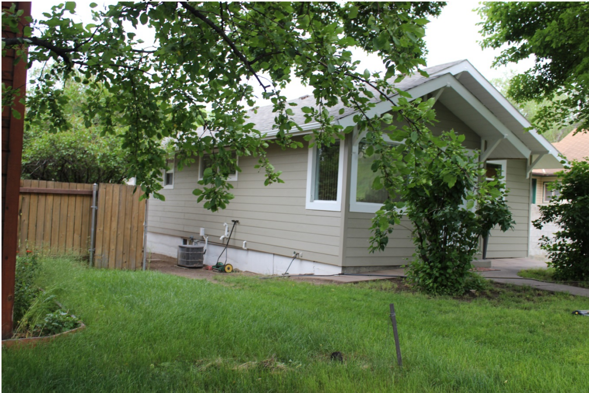
Photo Supplied by: Becki Miller, 2016. West and north elevations, view to southeast.
