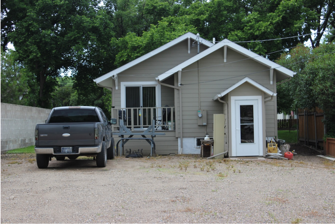
Photo Supplied by: Becki Miller, 2016. East (rear) elevation, view to west.
