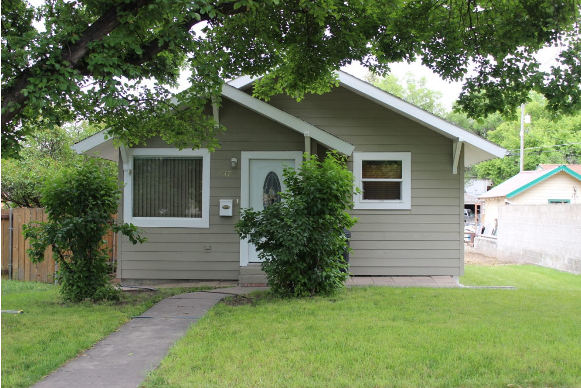
Photo supplied by: Becki Miller, 2016. West (front) elevation, view to the east.
