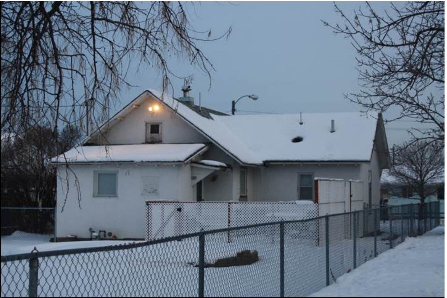
View to northeast, 1068 N Ewing west elevation
