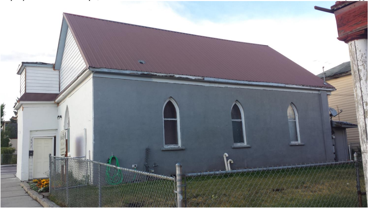
Shaffer's Chapel South Elevation, facing northeast 7/11/15 Photograph by Anthony Wood
