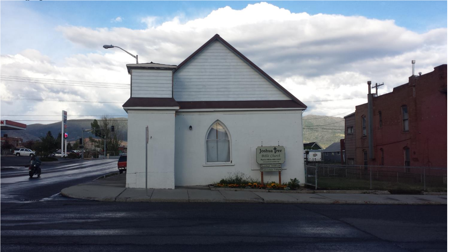
Shaffer's Chapel West façade, facing east 7/11/15 Photograph by Anthony Wood
