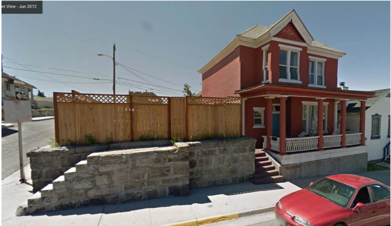
East-North Elevations – Photo Credit Google Maps
