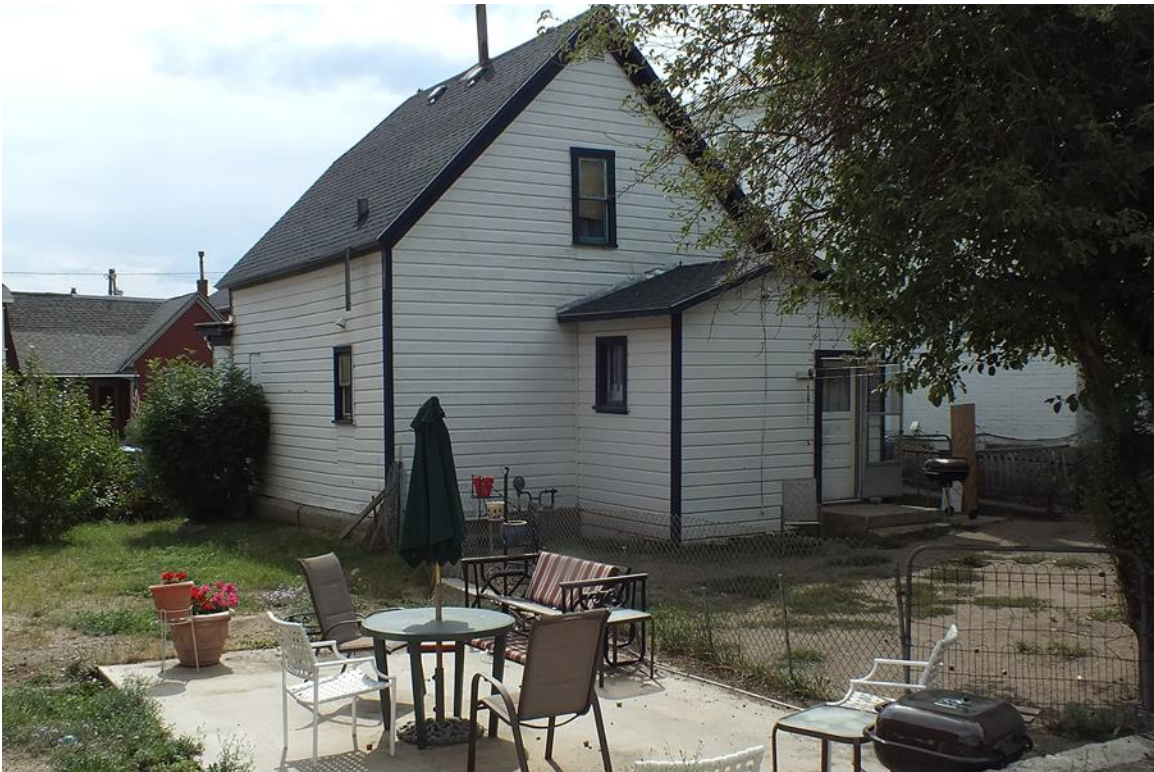
Walter and Alyce Duncan Residence, 711 West Broadway, Butte View to southwest, showing north (rear) and east elevations. Photo by Mary McCormick, 2016.
