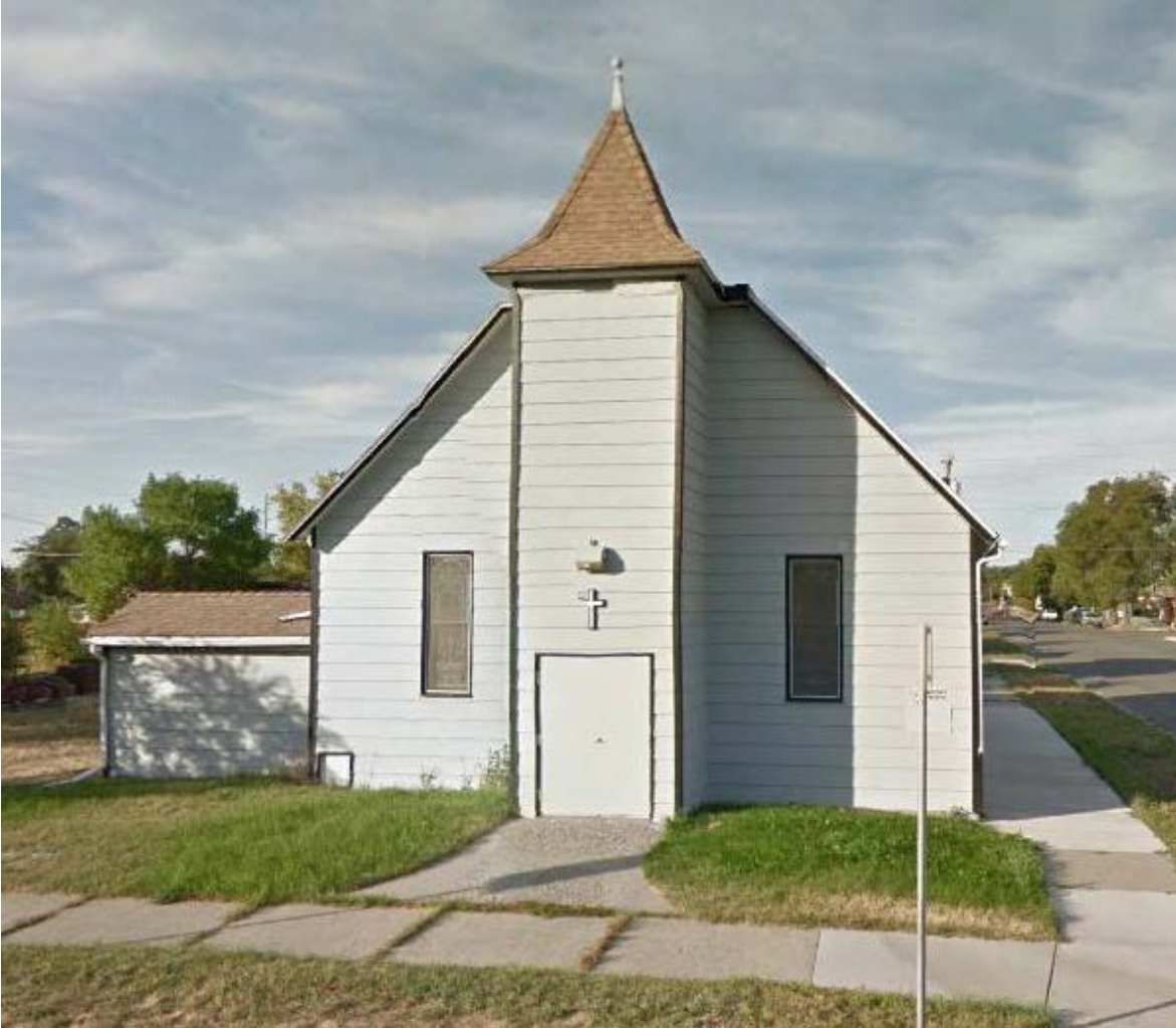
Wayman Chapel Northeast Façade, facing Southwest 8/13/15, (Google Earth Photo)
