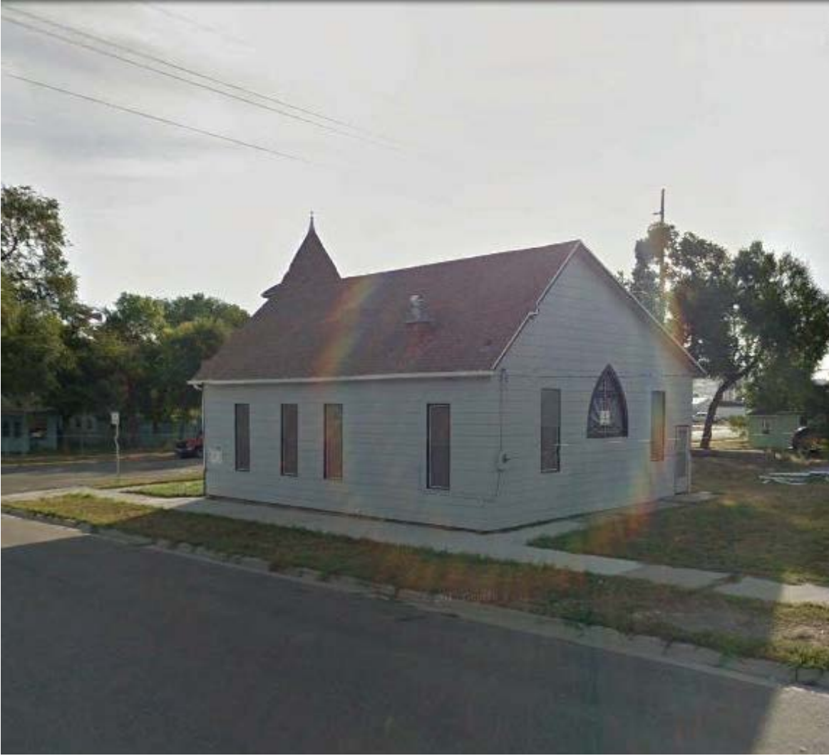
Wayman Chapel Northwest and Southwest elevations, facing east 8/13/15, (Google Earth Photo)
