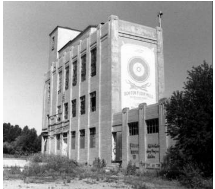
Figure 14. General Mills Elevator, Harlowton.
