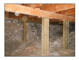
Thought the stabilizing timbers are in good shape, this is a temporary solution to an eminent problem that will eventually arise within all unreinforced stone structures in Virginia City.
