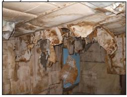
No south interior wall remains in the Coggswell Cabin to shelter it from the elements, and the protective muslin covering what walls are left is clearly beyond repair with weather and water damage. This building is close to being classified as "Failed."
