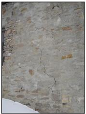
A view of the bowed out interior wall, and the exterior wall of the Montana Post building: Cracks are already appearing on the outside above where the section of stone has failed in the basement.
