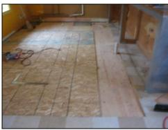
A broken hot water heater damaged the floor, causing the joists to rot. It was removed, and a new floor was put in its place.
