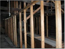
Though the clapboard false-front was preserved in 2009, the interior still retains the same temporary bracing that was placed in 2000 holding the roof up. This building was a display prior to the attempt at full stabilization, and the collections removed from the Prasch have put a strain on already overcrowded storage facilities.
