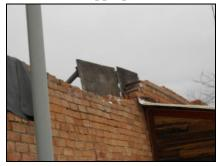
Rubber sheeting and plywood buttresses are employed to keep the brick parapet from collapsing all-together. These are temporary measures until the problem can be addressed with masonry.
