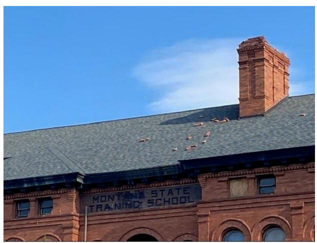
Damage caused by a windstorm in January, 2021. The chimney cover was blown off and several bricks have been damaged.
