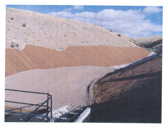
Figure 3. Recently built flood mitigation pond and spillway up Hangman's Gulch at Bannack State Park.
