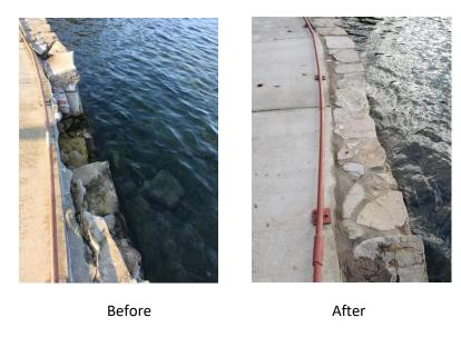
Figure 12: In-kind repairs of historic rockwork on the walkway at Roe Island, Giant Springs State Park.
