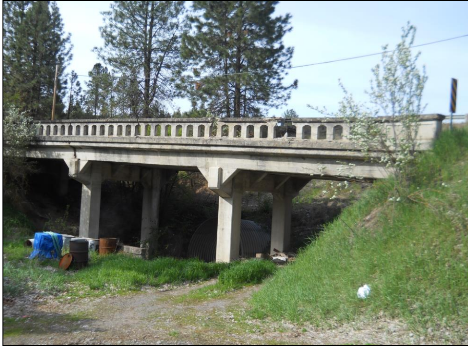
14-Mile (Nemoté) Creek Bridge (24MN0349) in Mineral County
