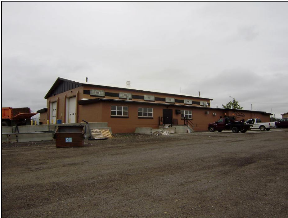
The Billings Air National Guard Building (24YL1996) now functions as the MDT’s Billings Maintenance Section Shop.
