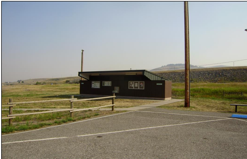
The restroom building at the Raynold’s Pass Rest Area in Madison County
