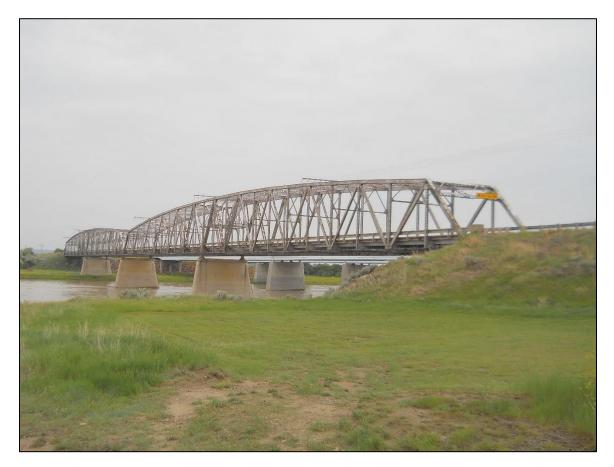
The Yellowstone River Bridge at Fallon is the most massive continuous span through truss in the state and a landmark in southeastern Montana. The bridge is listed in the National Register of Historic Places.
