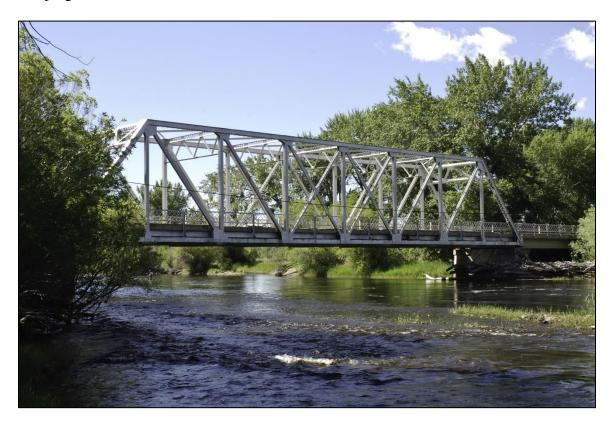
The Big Hole River/Kalsta Bridge (24BE2061/24MA2094), 22 miles north of Dillon, is an excellent example of a late 1920s highway department-designed through truss bridge.
