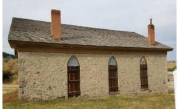
East Elevation: Stone masonry, unfinished wood windows, modified sliding wood door, decorative wood trim, and wood shingles.
