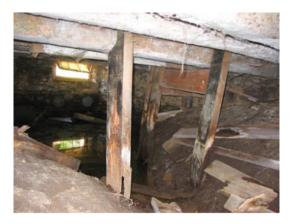
Figure 25: Gilbert House - basement subject to flooding leading to extensive interior moisture damage
