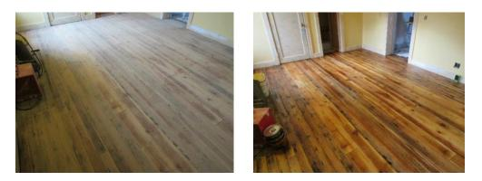
Figure 12: Harding House Interior - kitchen floor before and after refinishing
