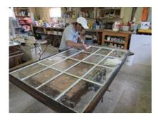
Figure 1: Sauerbier Blacksmith Shop window – The brittle nature of old wood makes window repair a slow and delicate operation.
