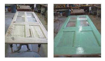
Figure 18: Smith Cabin - restore exterior doors; before and after
