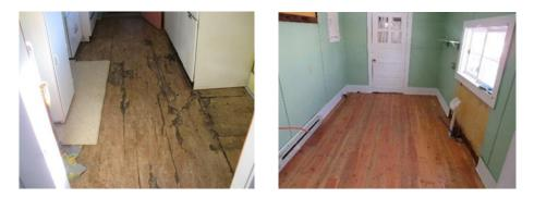
Figure 16: Smith Cabin - stabilize subfloor, install and finish new flooring; before and after
