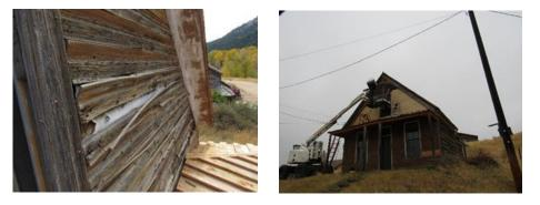
Figure 10: Harding House Exterior - siding replacement
