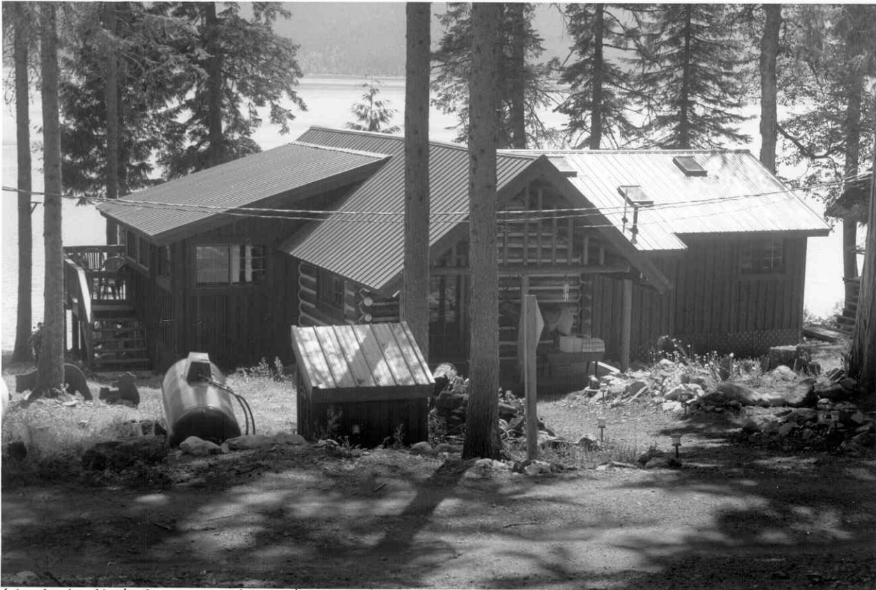
Cabin 6, Kelly's Camp Historic District Glacier National Park, Flathead County, Montana Photograph No. 11
