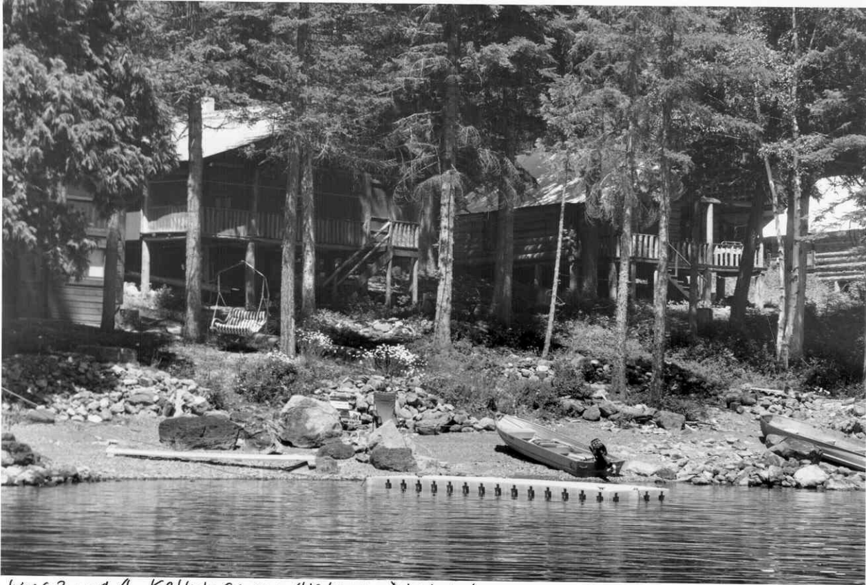
Cabins 3 and 4, Kelly's Camp Historic District Glacier National Park, Flathead County, Montana Photograph No. 8
