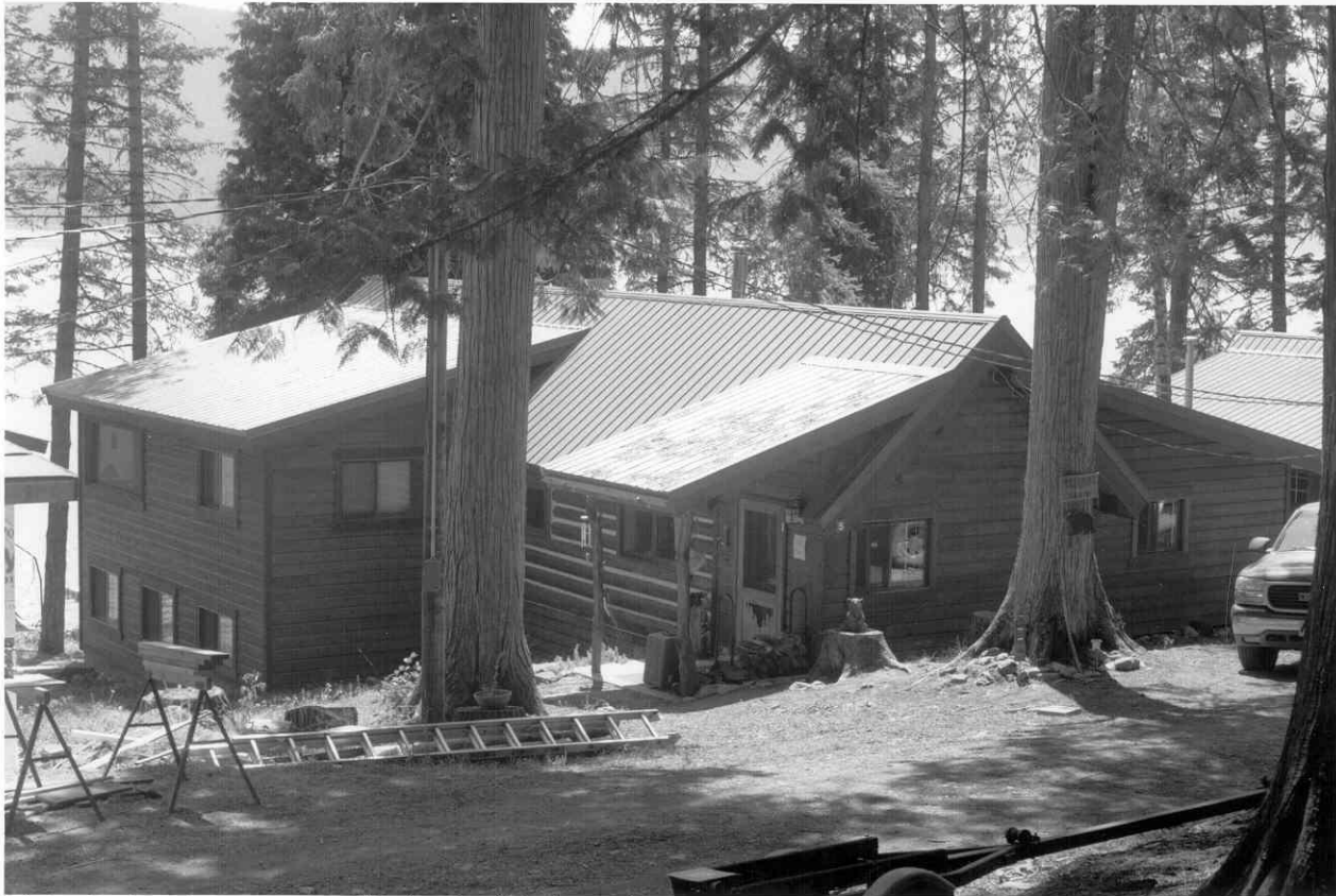
Cabin 5, Kelly's Camp Historic District Glacier National Park, Flathead County, Montana Photograph No. 10
