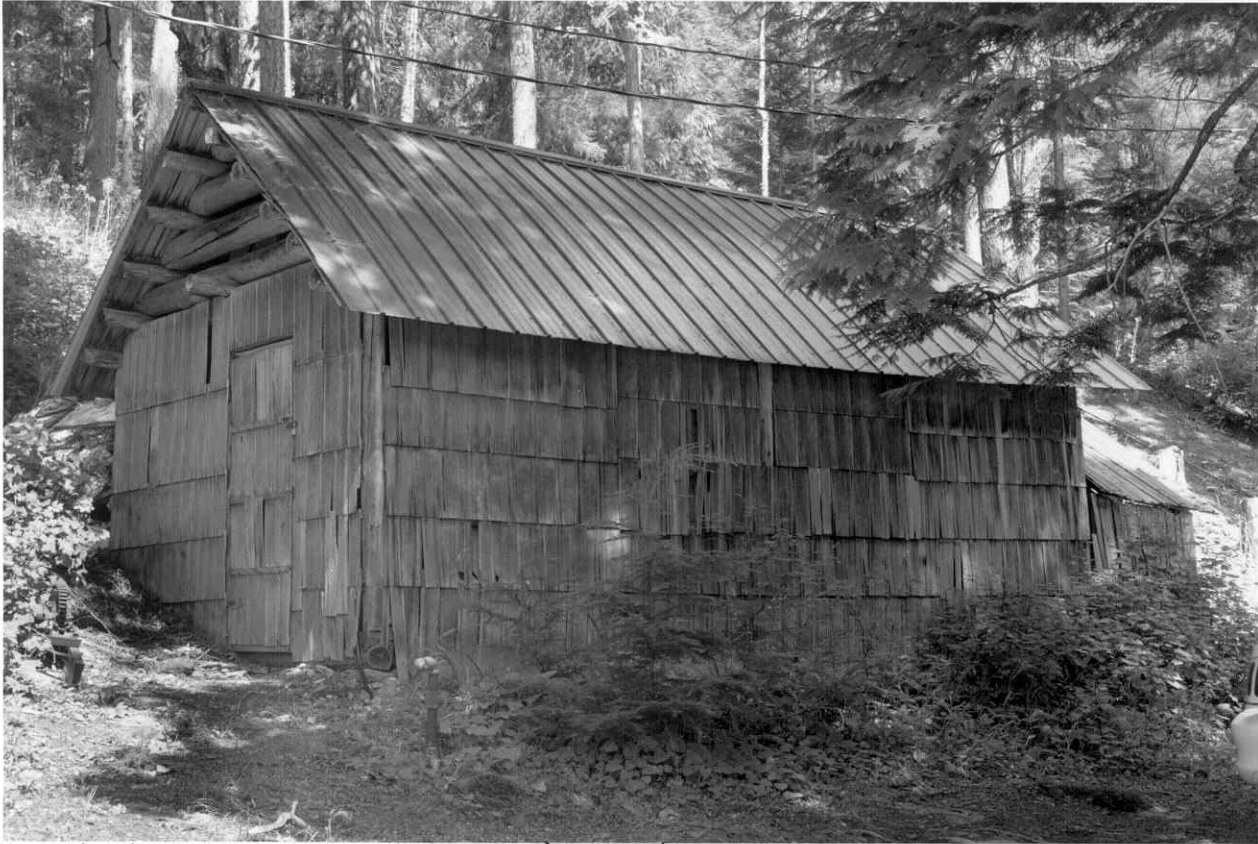
Woodshed, Kelly's Camp Historic District Glacier National Park, Flathead County, Montana Photograph No. 5
