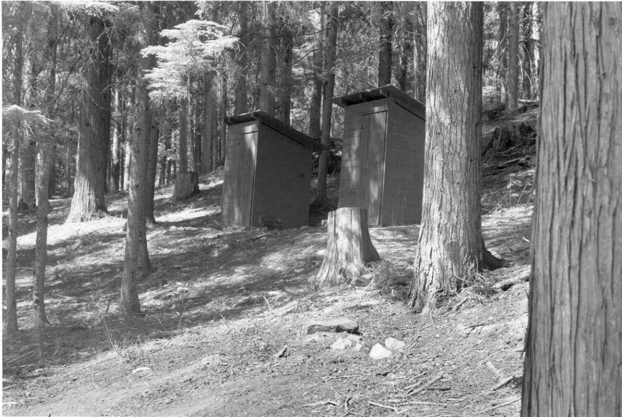
Privies behind Cabin 00, Kelly's Camp Historic District Glacier National Park, Flathead County, Montana Photograph No. 14
