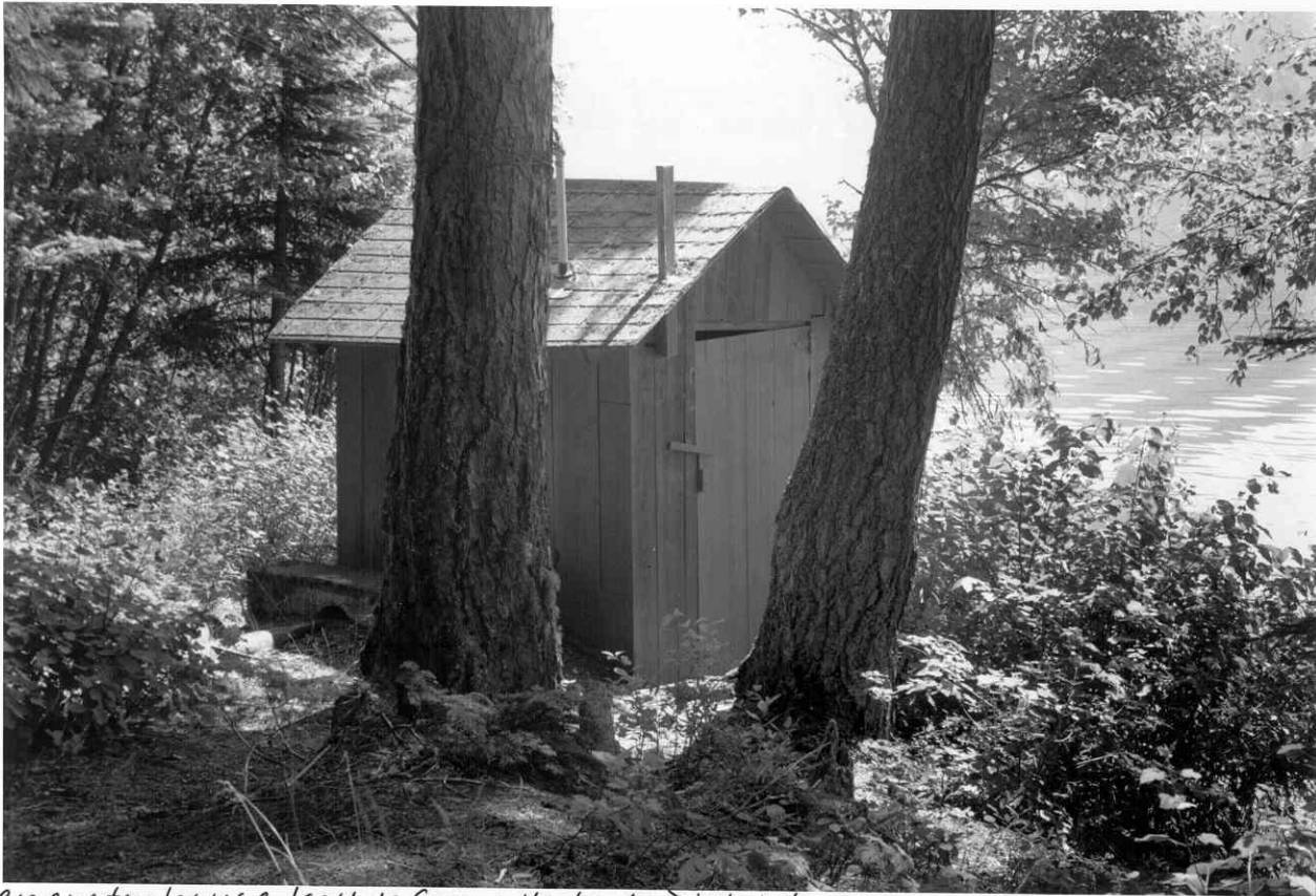
Generator house, Kelly's Camp Historic District Glacier National Park, Flathead County, Montana Photograph No.4
