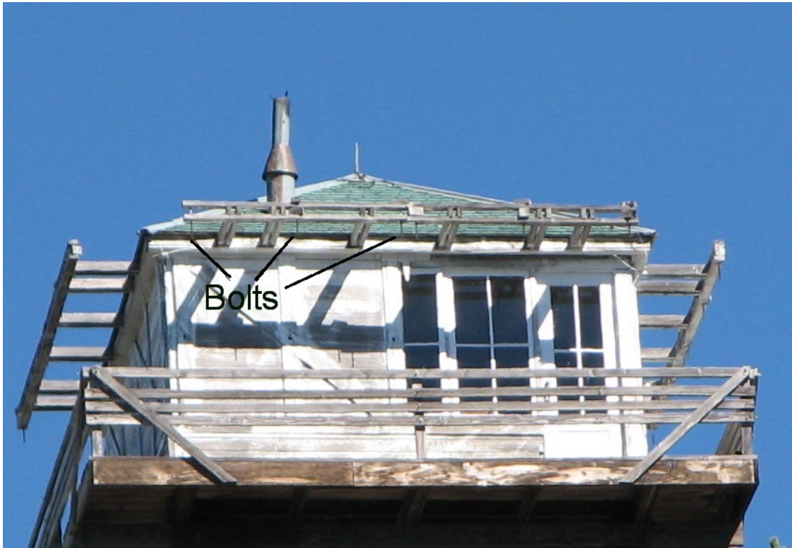
Figure 7. Mineral Peak Lookout on the Lolo National Forest: a modified L-4 plan with outriggers to hold shutters open (CRCS 2016).
