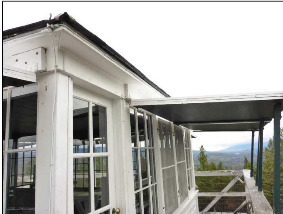
Figure 6. Double Arrow Lookout on the Lolo National Forest, an original 1931-plan with struts holding the shutters open (Sydney Bacon, 2016).
