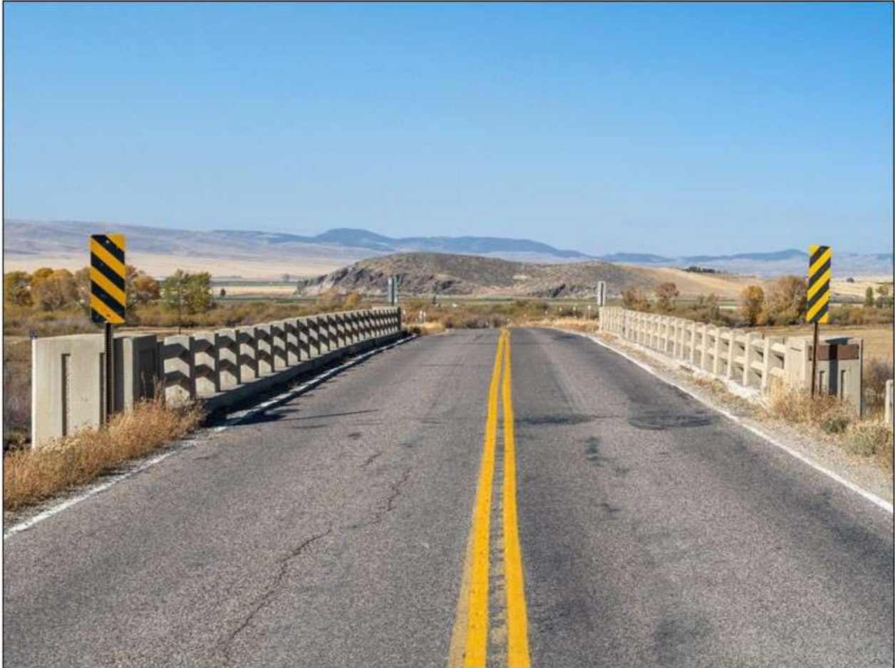
Oregon Short Line Overpass. East approach. View to the west. MT_BeaverheadCounty_BridgesOfPoindexterSloughHistoricDistrict_0015.
