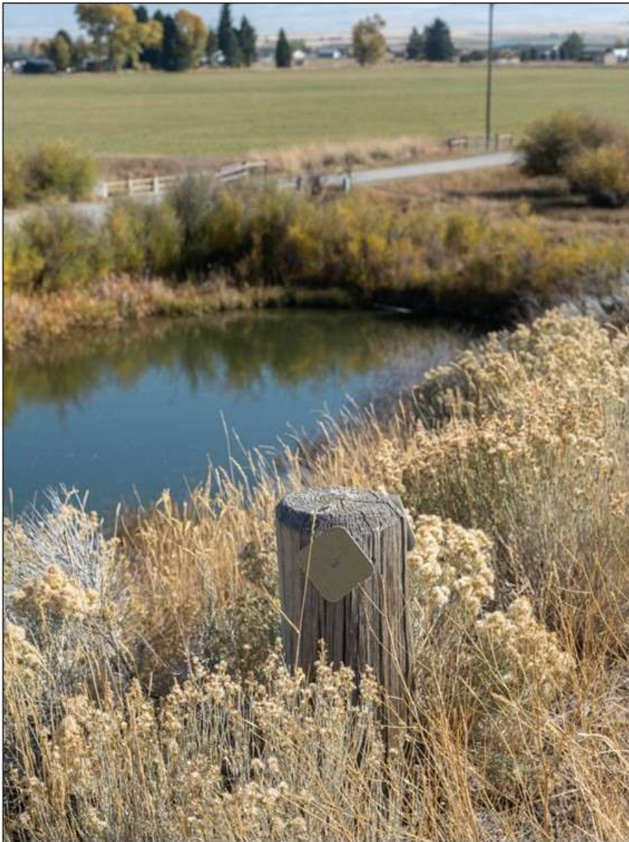
Montana Secondary 222/Old U.S. 91. Guard post detail. MT_BeaverheadCounty_BridgesOfPoindexterSloughHistoricDistrict_0025.
