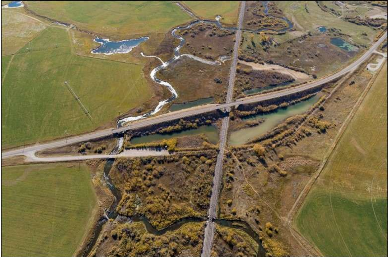
Bridges of Poindexter Slough Historic District. Overview. View to the south. MT_BeaverheadCounty_BridgesOfPoindexterSloughHistoricDistrict_0002.
