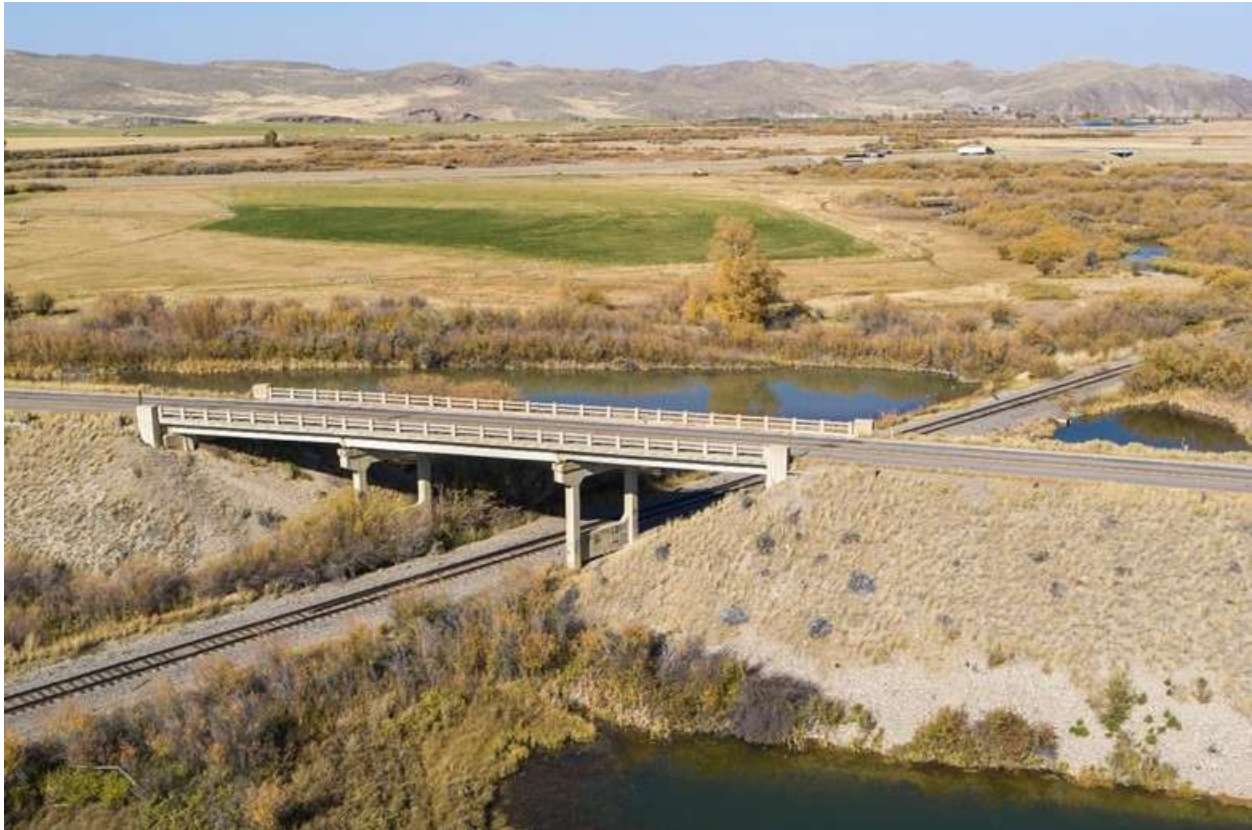
Oregon Short Line Overpass. Overview. South side. View to the northwest. MT_BeaverheadCounty_BridgesOfPoindexterSloughHistoricDistrict_0011.
