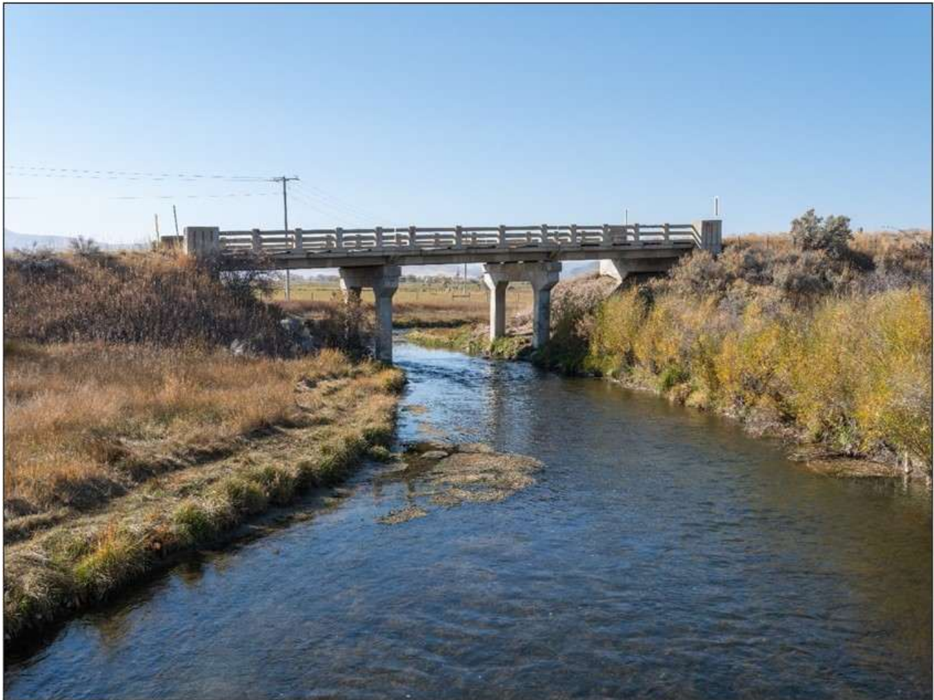
Poindexter Slough Bridge. North side. View to south. MT_BeaverheadCounty_BridgesOfPoindexterSloughHistoricDistrict_0006.
