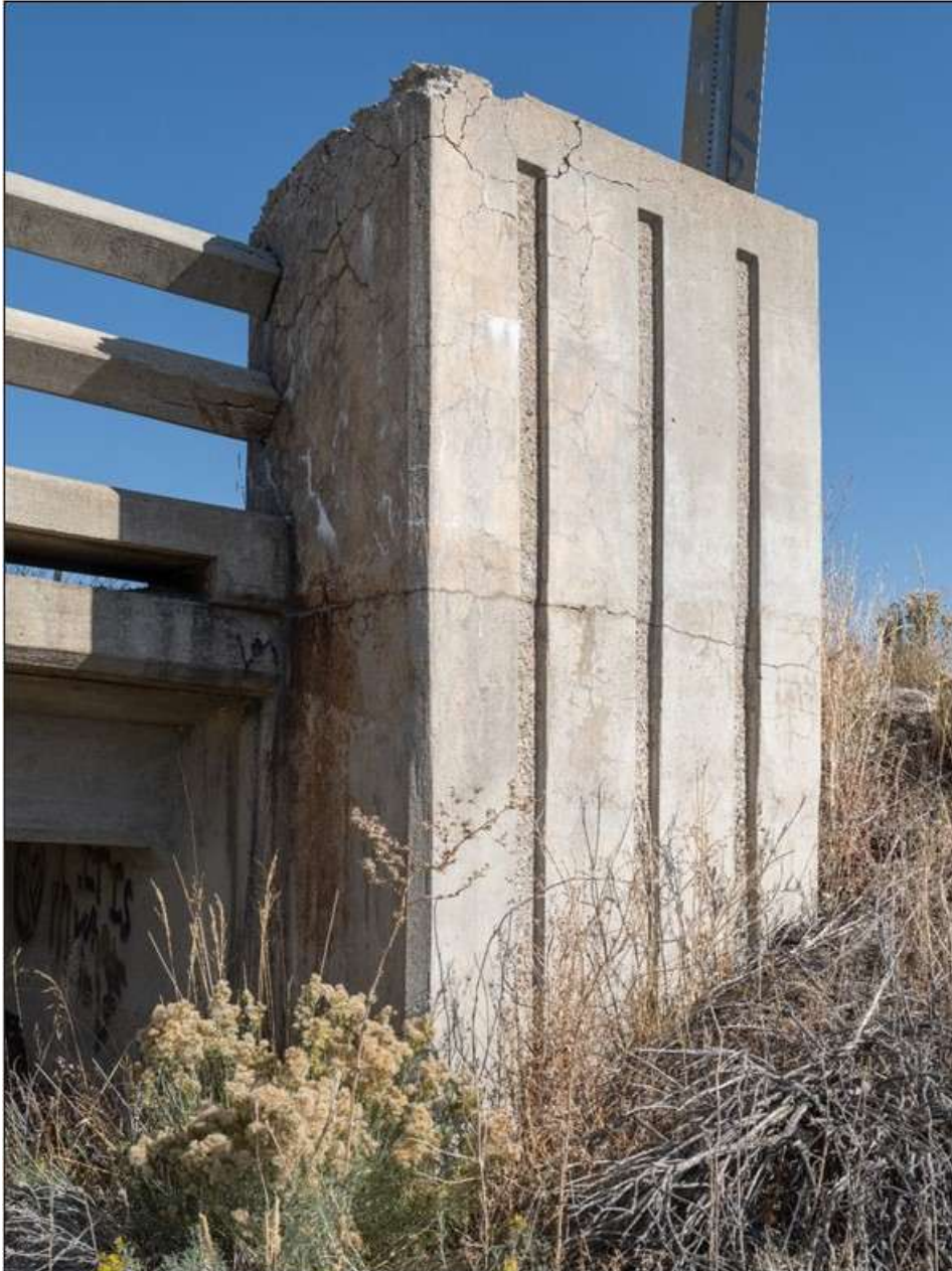
Poindexter Slough Bridge. Detail of endpost. MT_BeaverheadCounty_BridgesOfPoindexterSloughHistoricDistrict_0009.
