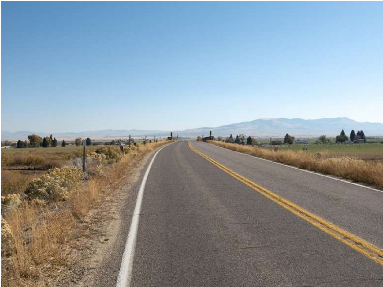
Montana Secondary 222/Old U.S. 91. View to west. MT_BeaverheadCounty_BridgesOfPoindexterSloughHistoricDistrict_0019.
