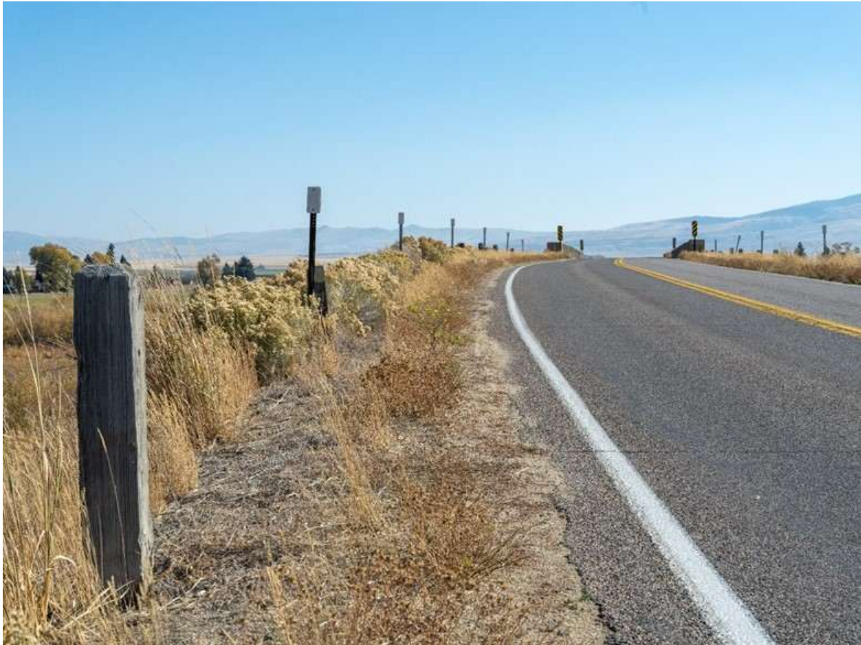
Montana Secondary 222/Old U.S. 91. Detail of guard posts. View to east. MT_BeaverheadCounty_BridgesOfPoindexterSloughHistoricDistrict_0022.
