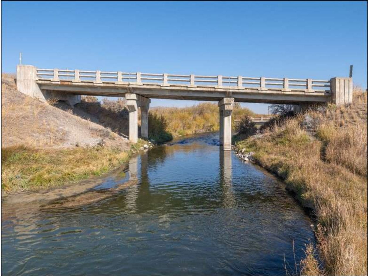
Poindexter Slough Bridge. South side. View to north. MT_BeaverheadCounty_BridgesOfPoindexterSloughHistoricDistrict_0004.
