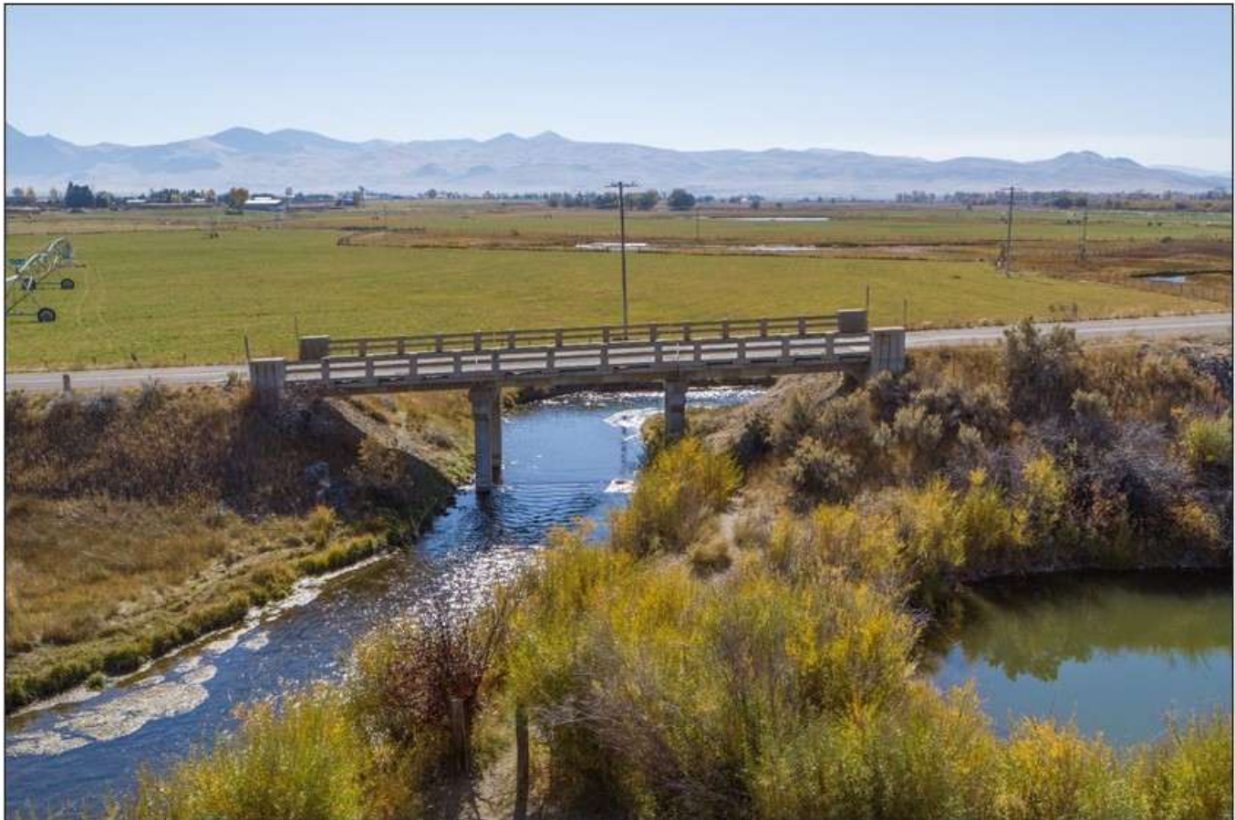
Poindexter Slough Bridge. North side. View to the south. MT_BeaverheadCounty_BridgesOfPoindexterSloughHistoricDistrict_0007.
