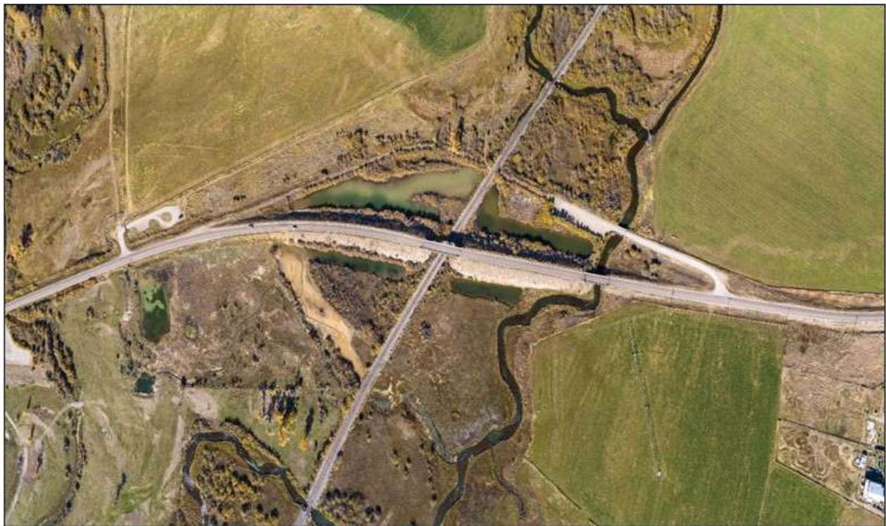
Bridges of Poindexter Slough Historic District. Overview. View to north. MT_BeaverheadCounty_BridgesOfPoindexterSloughHistoricDistrict_0001
