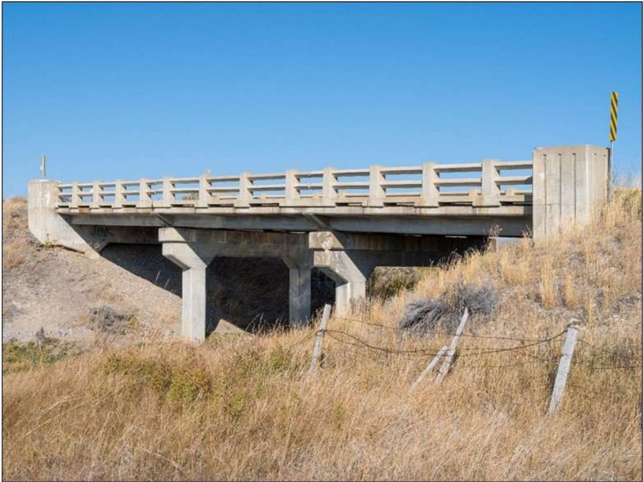
Poindexter Slough Bridge. South side. View to the northwest. MT_BeaverheadCounty_BridgesOfPoindexterSloughHistoricDistrict_0005.
