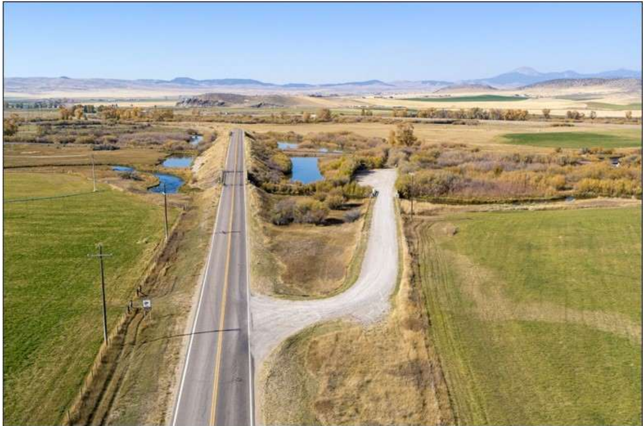
Old U.S. 91 alignment. View to west. MT_BeaverheadCounty_BridgesOfPoindexterSloughHistoricDistrict_0028.
