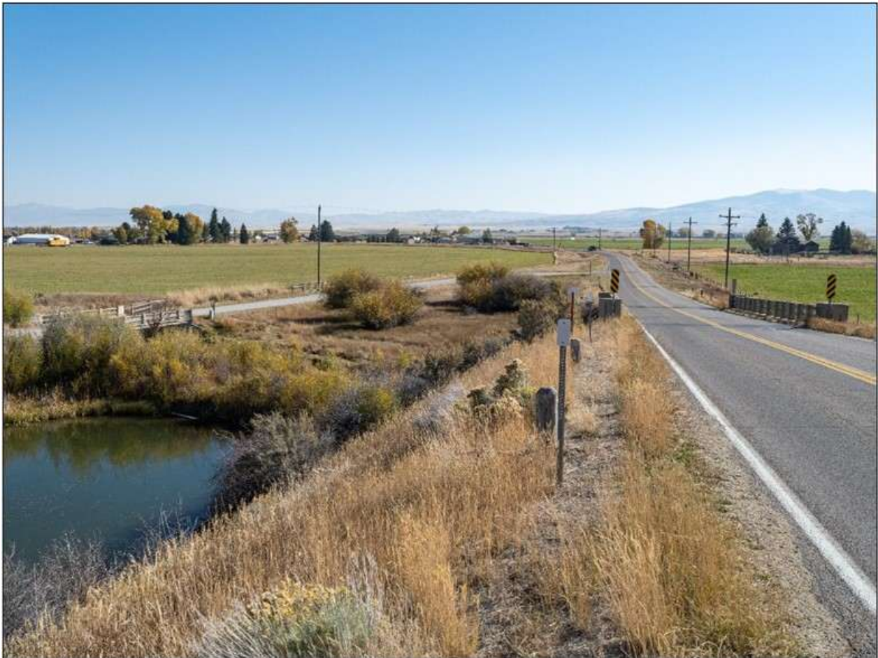
Montana Secondary 222/Old U.S. 91. Detail of guard posts. View to east. MT_BeaverheadCounty_BridgesOfPoindexterSloughHistoricDistrict_0024.
