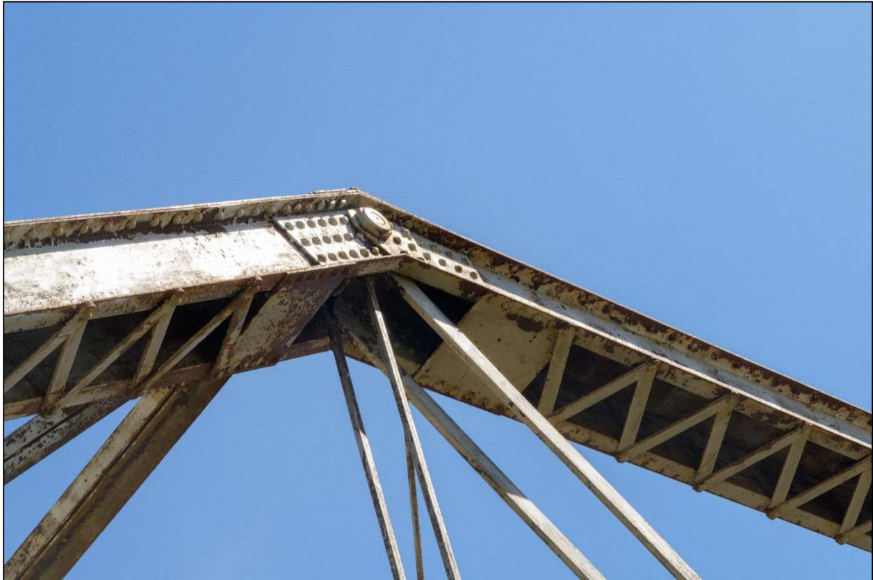
Milk River Bridge. Detail of upper chord and pin-connection. View to the north. MT_PhillipsCounty_MilkRiverBridge_0011.
