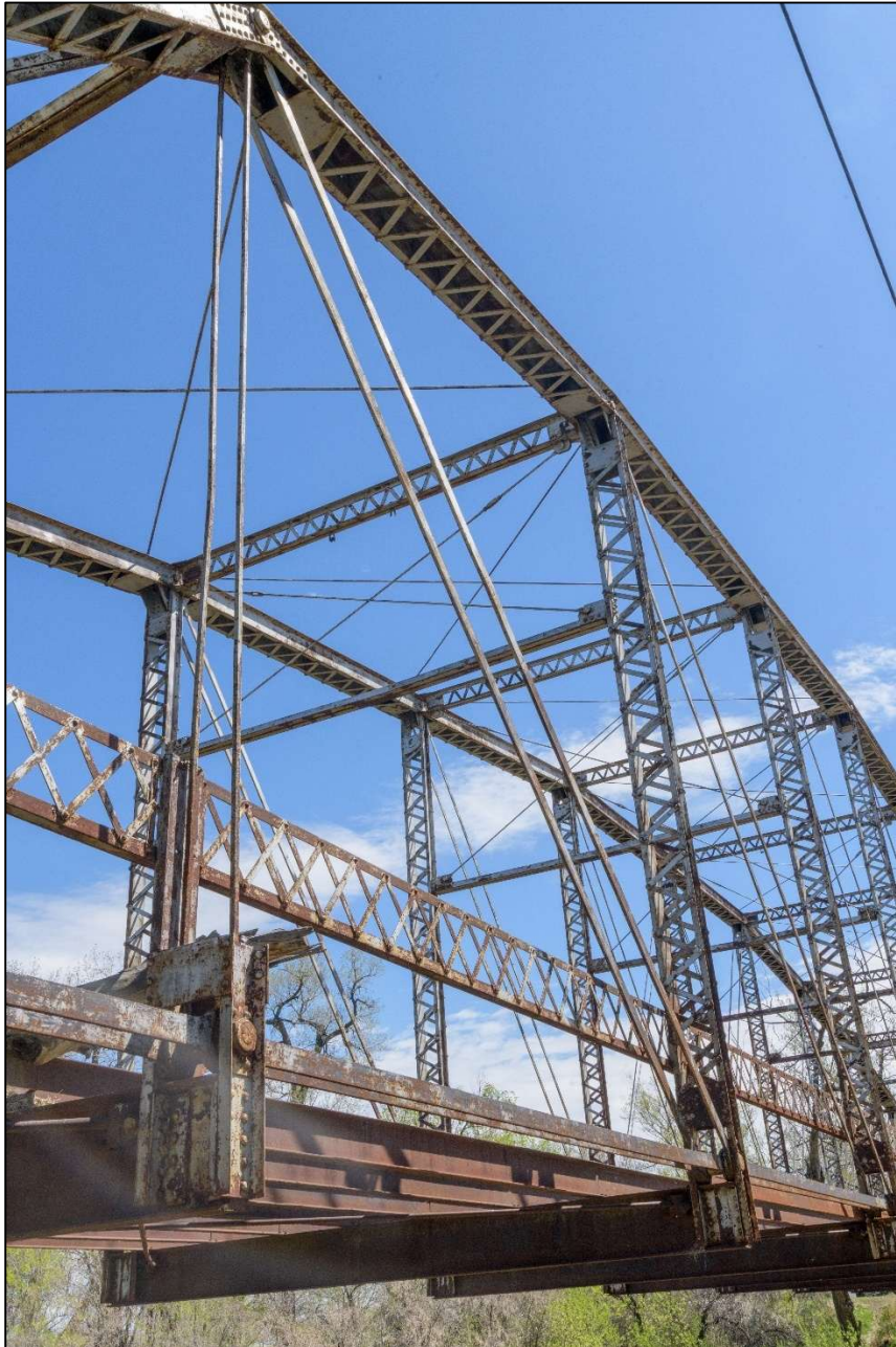
Milk River Bridge. Detail of Parker through truss and floor system. MT_PhillipsCounty_MilkRiverBridge_0010.
