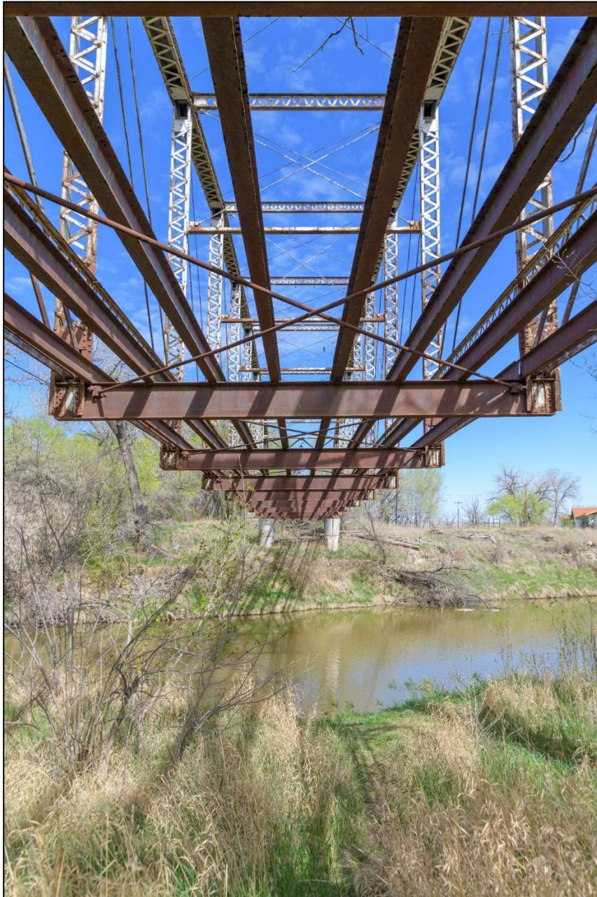
Milk River Bridge. Detail of stringers and floor beams. View to the northwest. MT_PhillipsCounty_MilkRiverBridge_0012.
