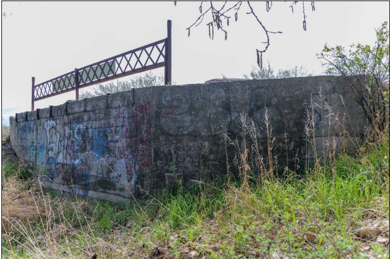
Milk River Bridge. Detail of southeast abutment and re-use of guard panel. View to southwest.
