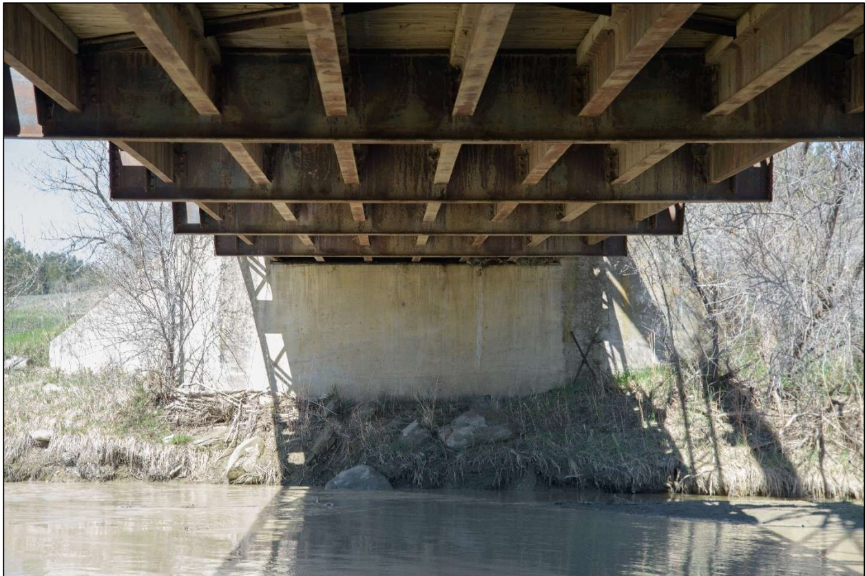
Musselshell River Bridge. detail of stringers and floor beams. View to the northwest. MT_GoldenValleyCounty_MusselshellRiverBridge_0010.
