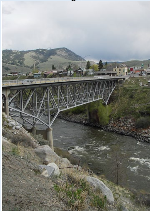
Gardiner Bridge, Gardiner
