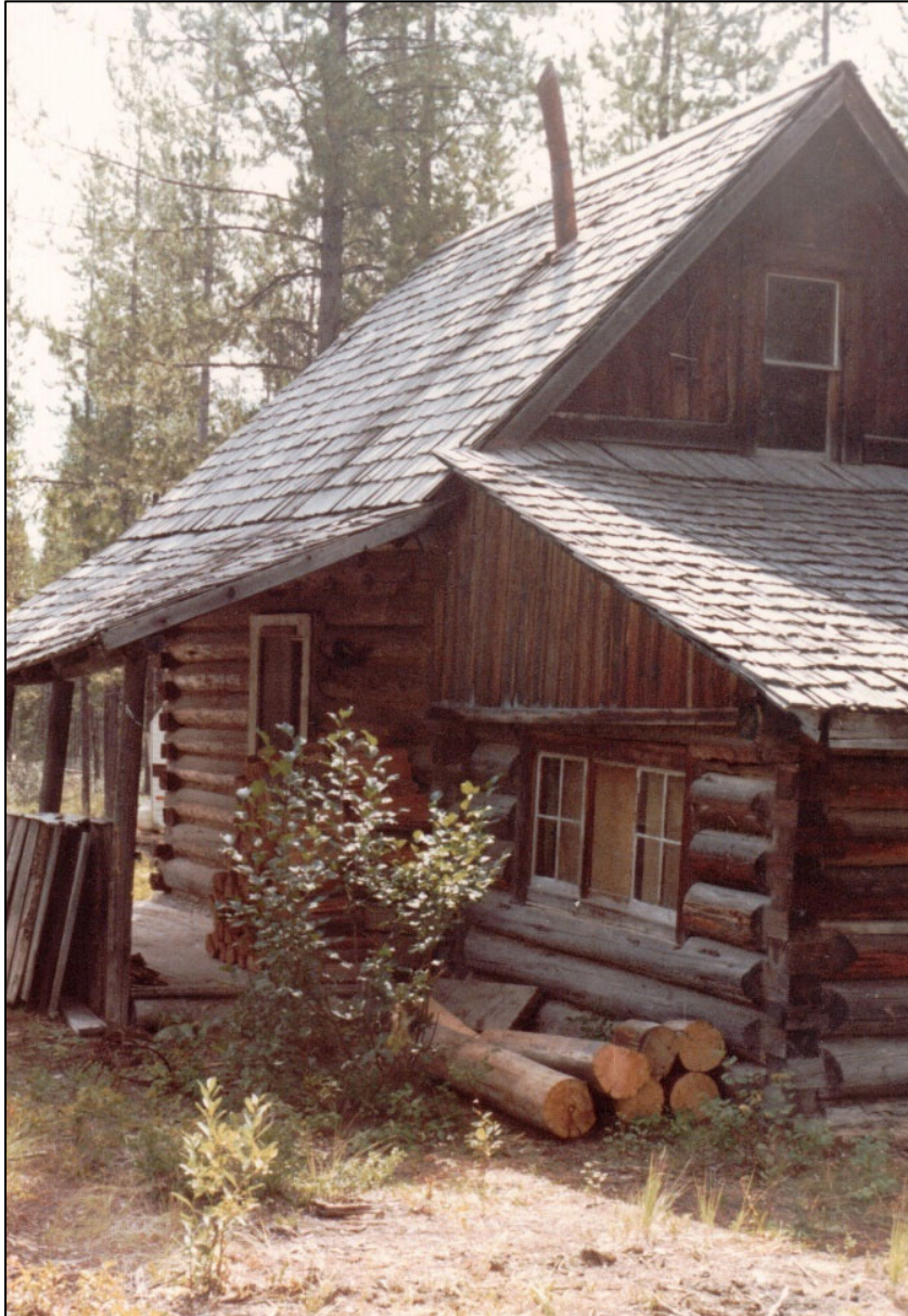
Billy Kruse Cabin, 1969. Cabin, showing 1929 addition, and porch from west. Photographer, Larry Wilson.
