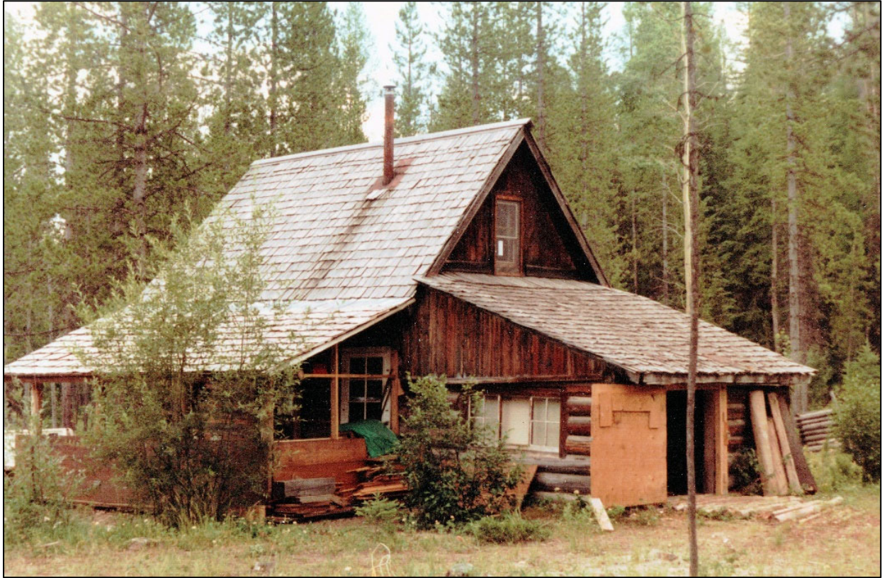
Billy Kruse Cabin, 1982. Cabin from northwest, view to southeast. Photographer, Larry Wilson.
