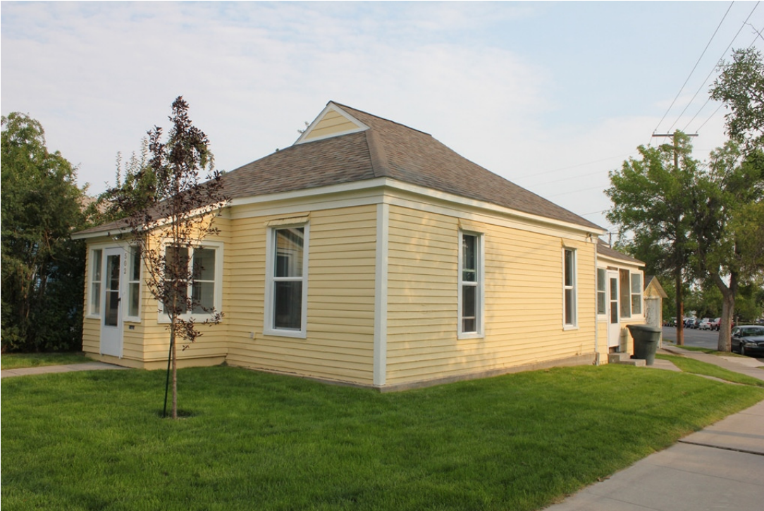
Haight - Bridgewater House, south and west elevations. View to northeast. 0002 of 0007.
