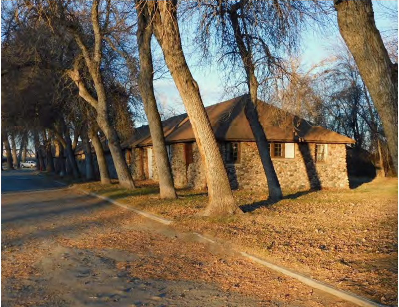
MT_YellowstoneCounty_RiversidePark_0031. Laurel Rifle Club long building, looking west / northwest. December 21, 2023.
