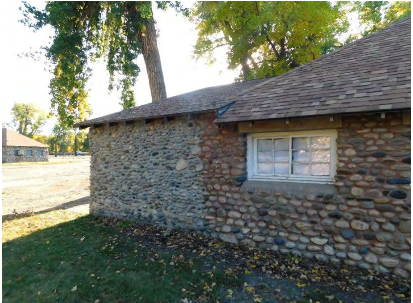
MT_YellowstoneCounty_RiversidePark_0013. American Legion Hall / Bath House, looking southwest at add-on façade from the 1950s (left) marked by color change in mortar. October 07, 2023.
