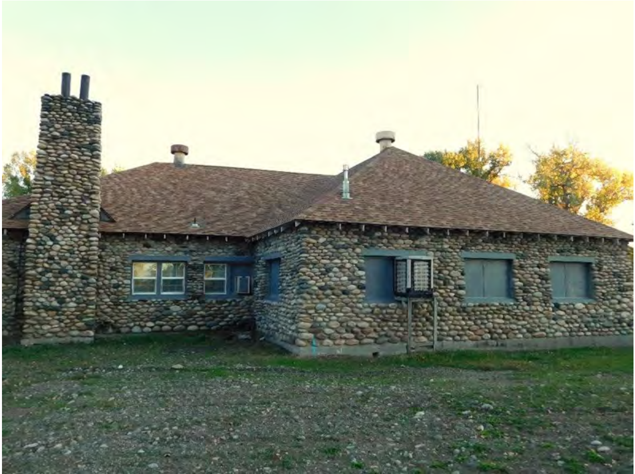
MT_YellowstoneCounty_RiversidePark_0003. Riverside Hall / Jaycee Hall, looking south. October 07, 2023.
