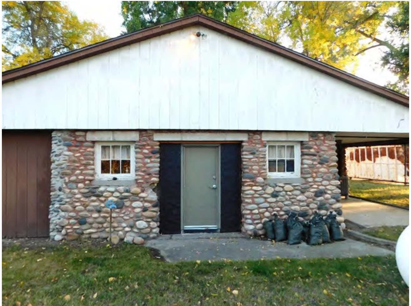
MT_YellowstoneCounty_RiversidePark_0015. American Legion Hall / Bath House, looking south. The back façade in photograph faces the Yellowstone River. October 07, 2023.
