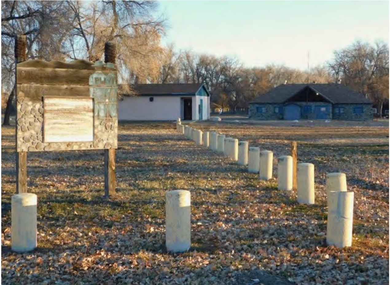
MT_YellowstoneCounty_RiversidePark_0027. World War II Prisoner of War sign at entrance to Riverside Park, with concrete restroom and Riverside Hall / Jaycee Hall in the background, looking east / northeast. December 21, 2023.
