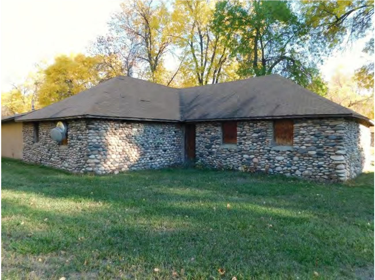
MT_YellowstoneCounty_RiversidePark_0018. Rifle Club building, view looking southeast. Northwest corner of the long building. October 07, 2023.
