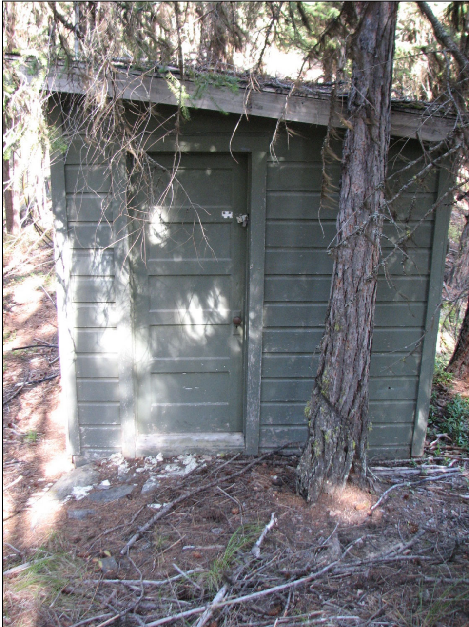
MT_MineralCounty_StRegisAirwayBeacon_0005. Warming shed. South side. View to the north.
