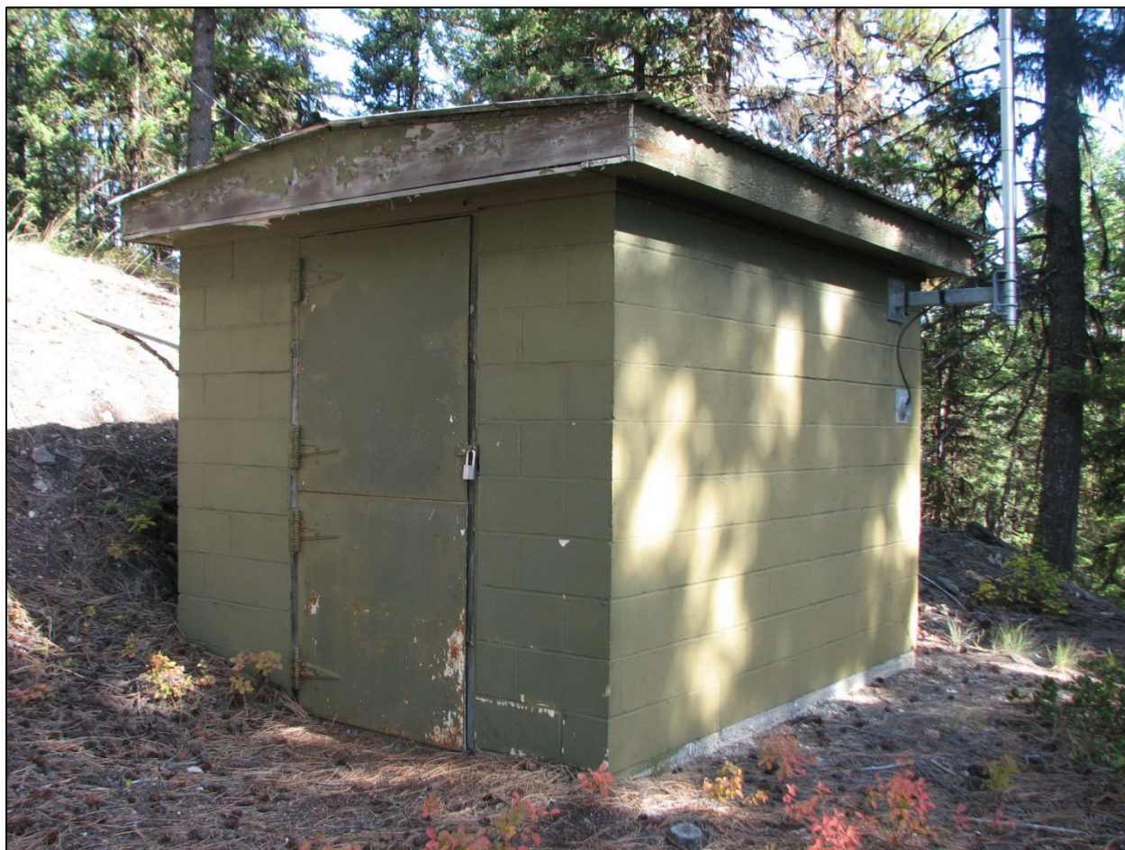
MT_MineralCounty_StRegisAirwayBeacon_0008. Electrical shed. West and south sides. View to the northeast.
