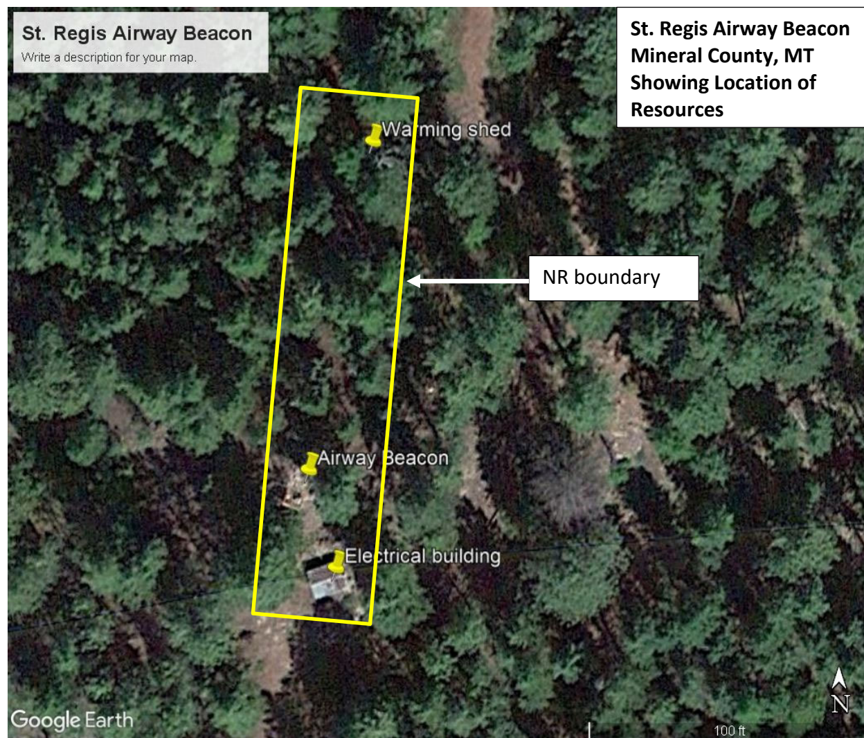
Location of St. Regis Airway Beacon, electrical shed, and warming shed, aerial view. Electrical building = Lat. 47.287107 Long. -115.050499 St. Regis Airway Beacon = Lat. 47.287192 Long. -115.050533 Warming shed = Lat. 47.287501 Long. -115.050425
