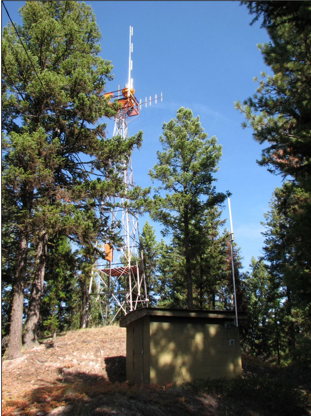
MT_MineralCounty_StRegisAirwayBeacon_0001. Overview. View to the northwest.
