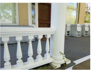
Picture 16: Porch balusters repaired, anchored &
