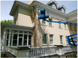
Picture 15: Roof trim being repaired & painted painted
