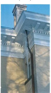
Picture 12: Before repair: Leaking gutters & downspouts
