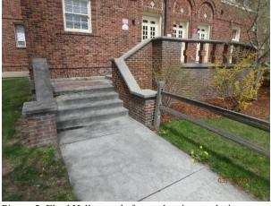
Picture 2: Elrod Hall steps: before – showing cracks in steps
