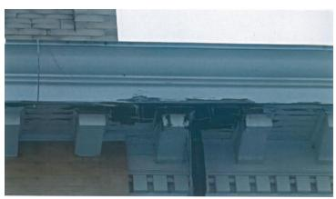
Picture 11: High roof trim & fascia before repair showing damage.
