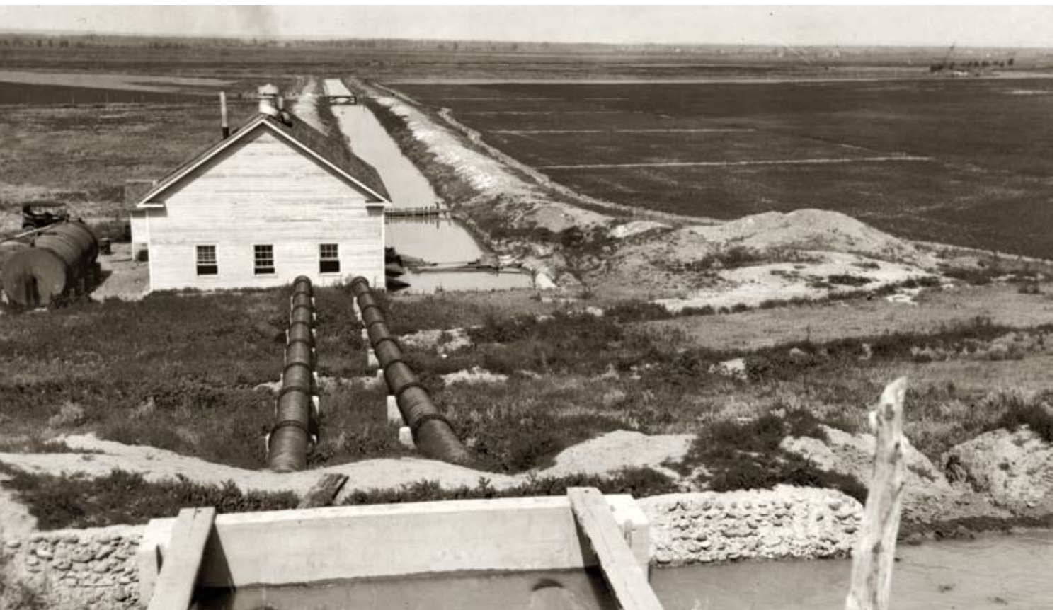
FIGURE 13.4: This pumping station lifts water into the irrigation canals of the Box Elder Irrigation District near Hysham. Irrigation projects were expensive and could help only small areas.
